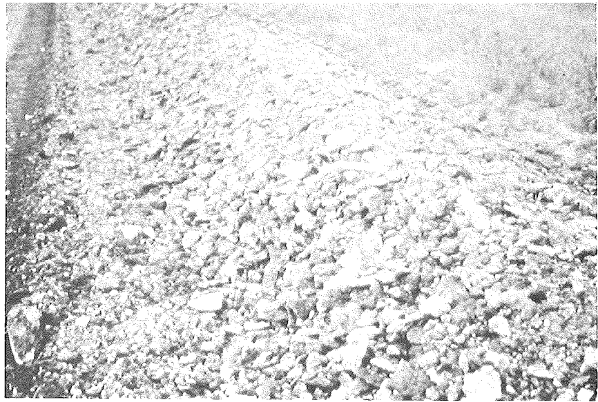
Windrow of crushed bituminous concrete from CMI Roto-mill.
