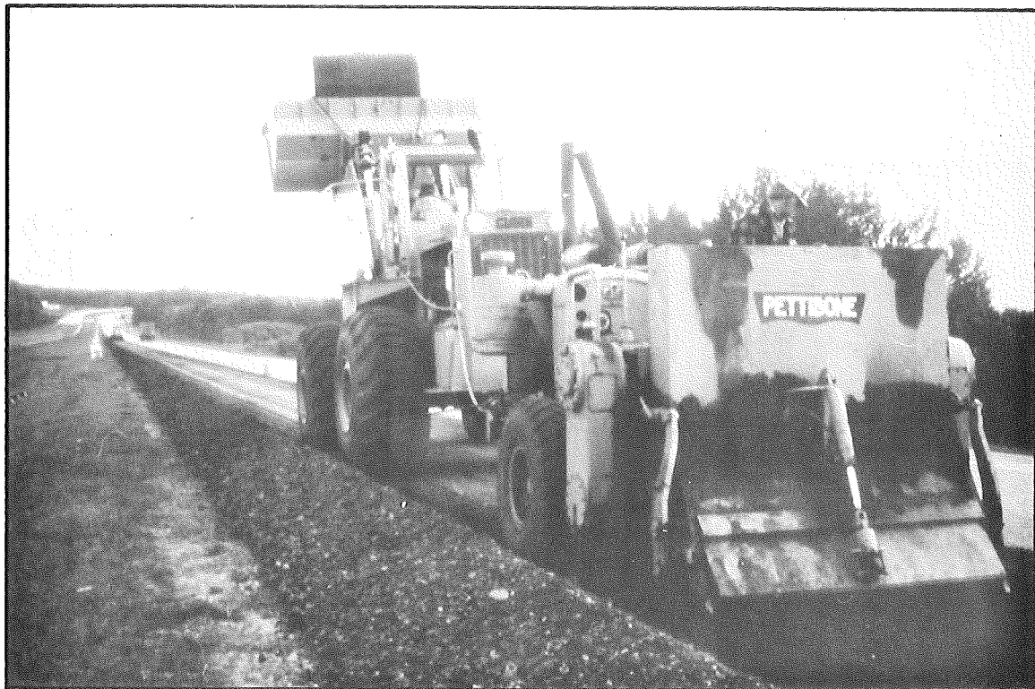
Pettibone hammermill crushing the remaining 2 in. of bituminous concrete.
