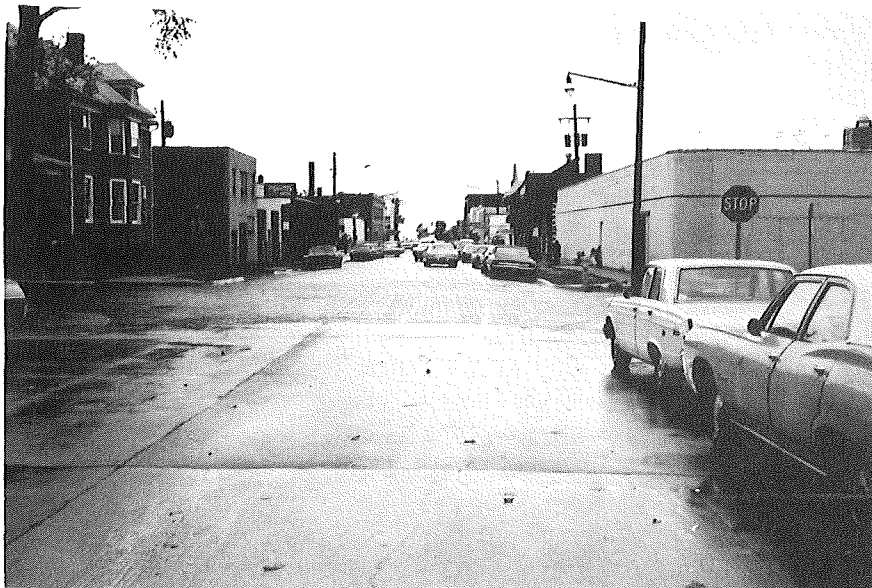
NORTHWESTBOUND PLEASANT STREET
