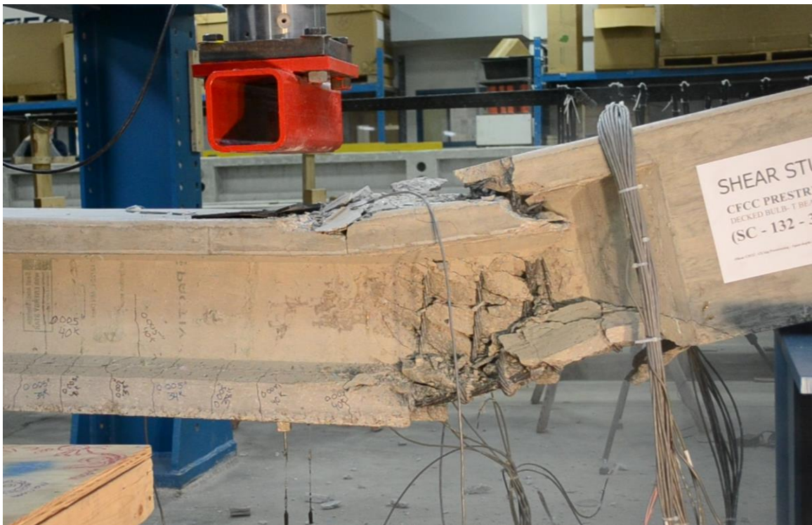
Figure 3.7-9 Beam C-C-S-B after failure
