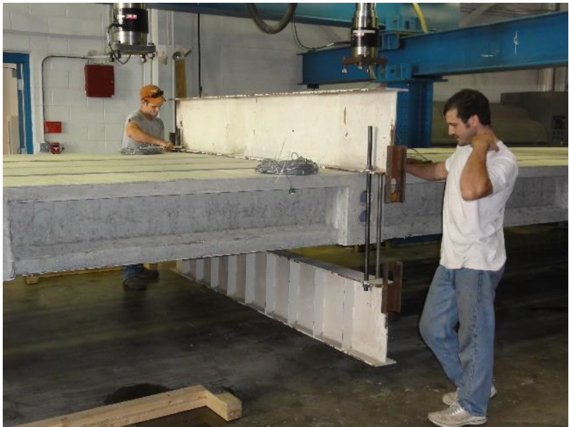
Figure 2.5-12 Beam leveling to eliminate differential camber
