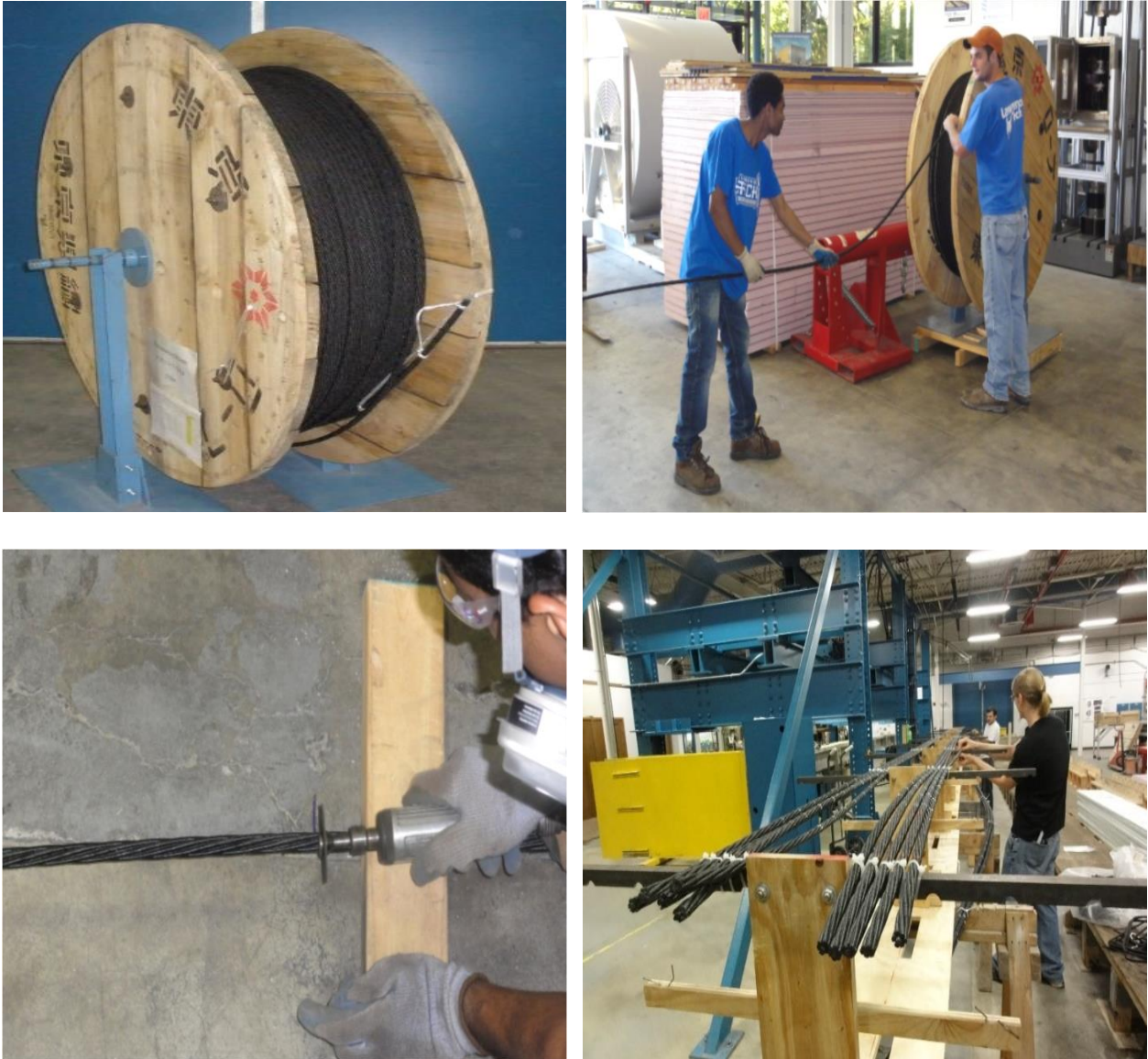
Figure 2.4-9 Cutting CFCC strands and constructing reinforcement cages
