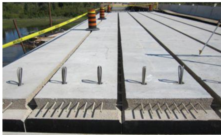
Figure 1.4-11 Construction of Eagle River Bridge, Ontario Canada
