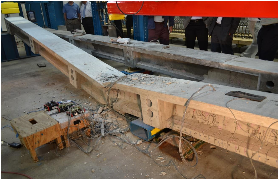
Figure 3.4-1 Beam C-S-F-O at failure
