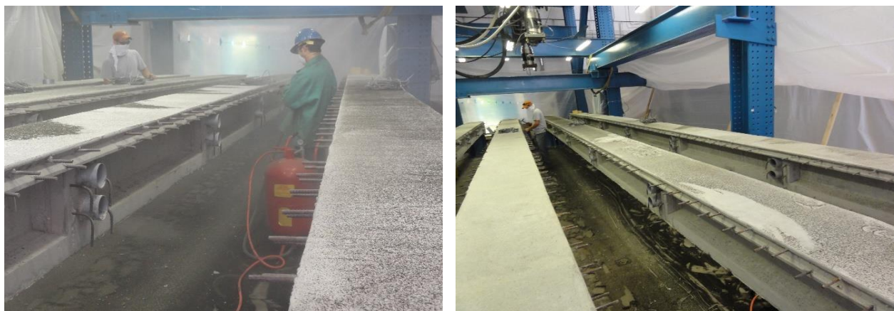
Figure 2.5-10 Sandblasting surfaces of the shear key joints
