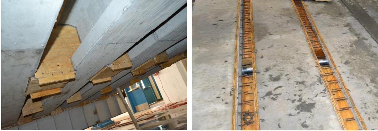
Figure 2.5-13 Formwork for shear key joints and around transverse diaphragms
