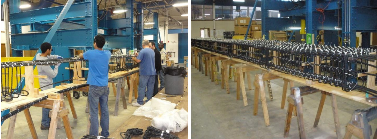
Figure 2.4-10 Building reinforcement cages for control beams
