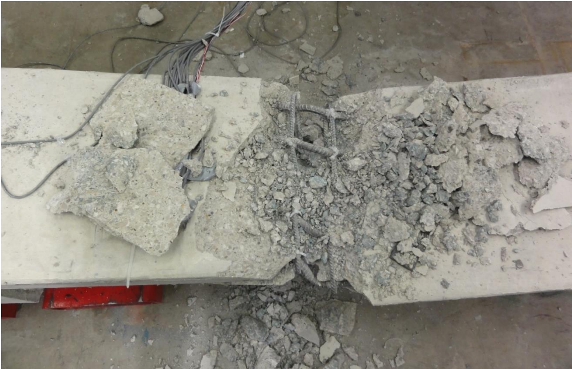
Figure 3.5-3 Buckling of top reinforcement in Beam S-S-F-U at failure
