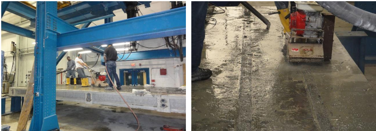
Figure 2.5-20 Grinding the surface of UHPC shear key joints
