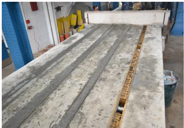
Figure 2.5-18 Pouring UHPC shear key joints
