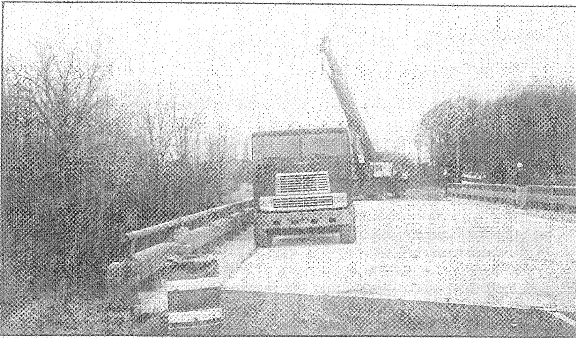
Figure 26: Truck position on day 1, position 1. (Trailer wheels adjacent to south curb.)
