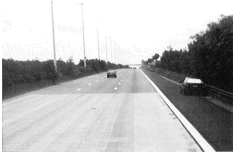
Figure 3.15 20-year-old CRCP in Belgium containing 0.85 percent reinforcement, AC interlayer, lean concrete base and a granular subbase. (Note that a portion was diamond ground to reduce noise emission of the original transverse tining).
