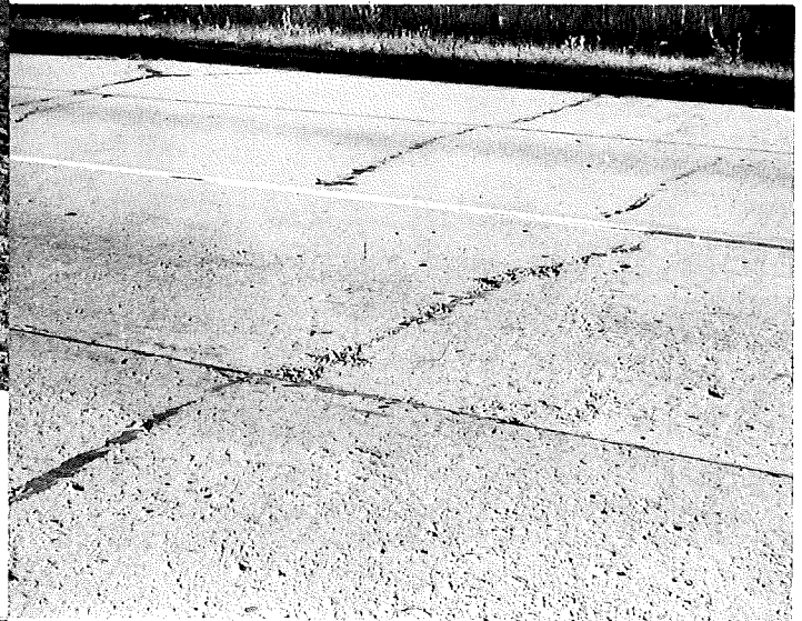
FIGURE 6. PATCHED AREA WITHIN PROJECT 21-28-C2 CONTAINING LIMESTONE AGGREGATE, CRACKED MUCH WORSE THAN OLDER BICHLER PAVEMENT. MORE RECENT THAN 19 YEAR OLD PROJECT.
