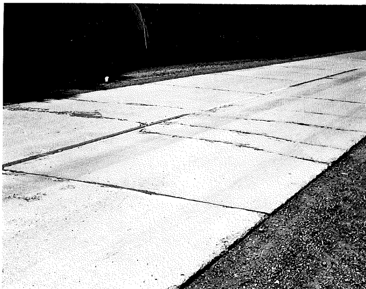
FIGURE 6. PATCHED AREA WITHIN PROJECT 21-28-C2 CONTAINING LIMESTONE AGGREGATE, CRACKED MUCH WORSE THAN OLDER BICHLER PAVEMENT. MORE RECENT THAN 19 YEAR OLD PROJECT.
