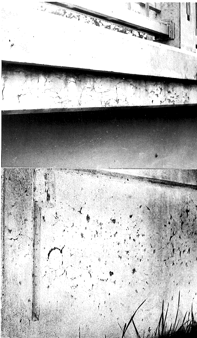
▲ FIGURES 8 AND 9. EXAMPLES OF YELLOW STAINED CRACKS IN BRIDGE SURFACES DUE TO LIMONITIC SANDSTONE IN IN COARSE AGGREGATE. B2 OF 21-9-12 AND B1 OF 21-14-2, BRIDGE 18 AND 19 YEARS OLD RESPECTIVELY.
