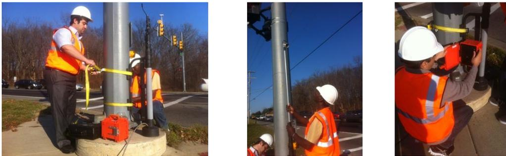
**Figure 4-1 Miovision Sensor Installation**
