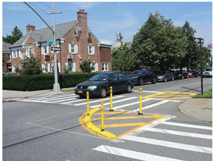
Figure 1. One-way to one-way parking removal and slow turn wedge treatment (Photo Credit: New York City DOT)
