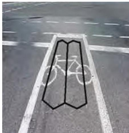
Figure 10. In-pavement bicycle loop detector
