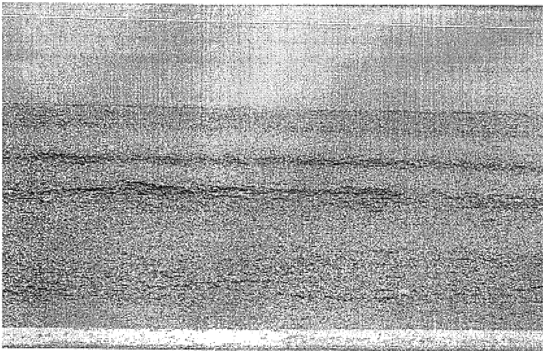
b) A close-up view of the segregated area in the passing lane
