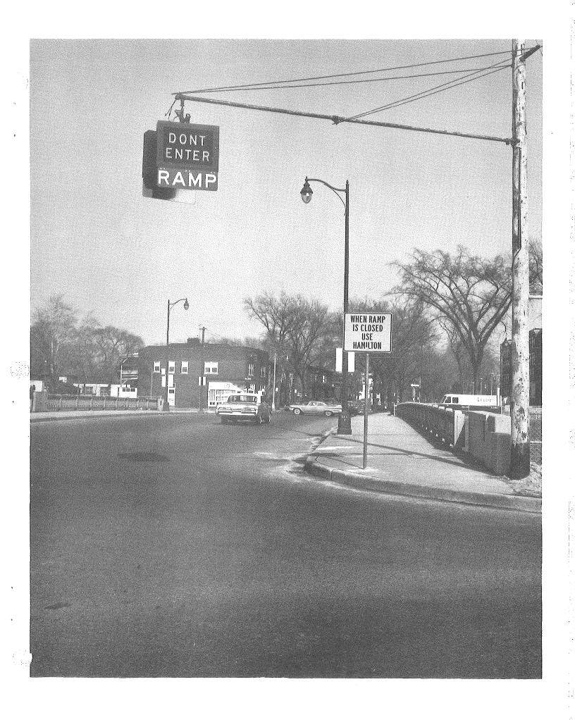
Preliminary tests to measure the effectiveness of the ramp signals were conducted in the spring of 1960. An experimental ramp signal was installed at the Trumbull Avenue entrance ramp to the westbound lanes of the Edsel Ford Freeway. The installation consisted of two back-to-back signals mounted on a mast arm so they would be visible to both directions of oncoming Trumbull Avenue traffic. The results of this experiment were documented in a paper by Richard D. Belprez and Conrad L. Dudek.
