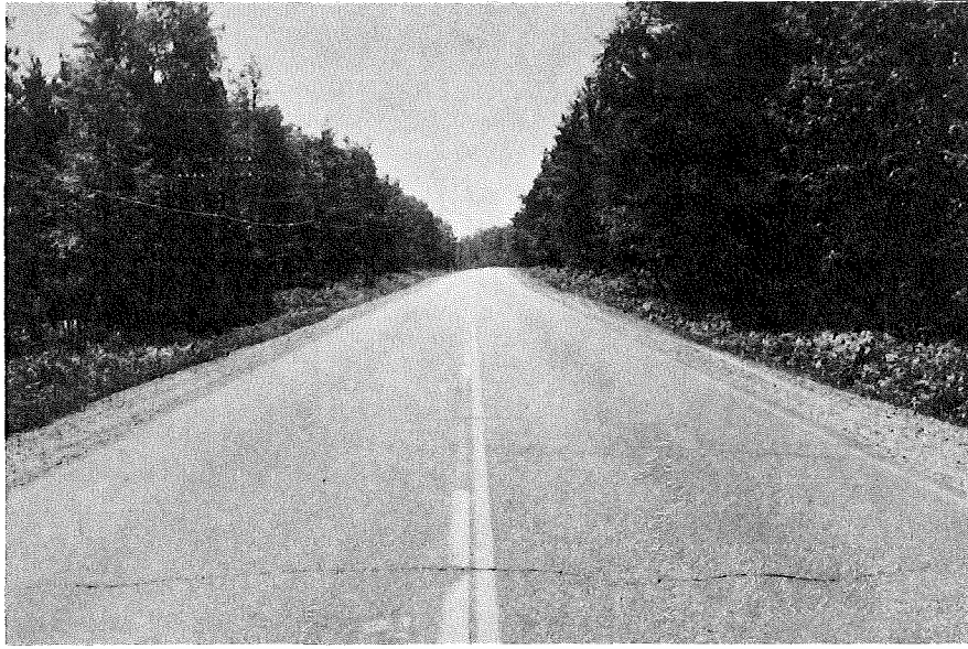
SOUTHBOUND CO. RD. 553
