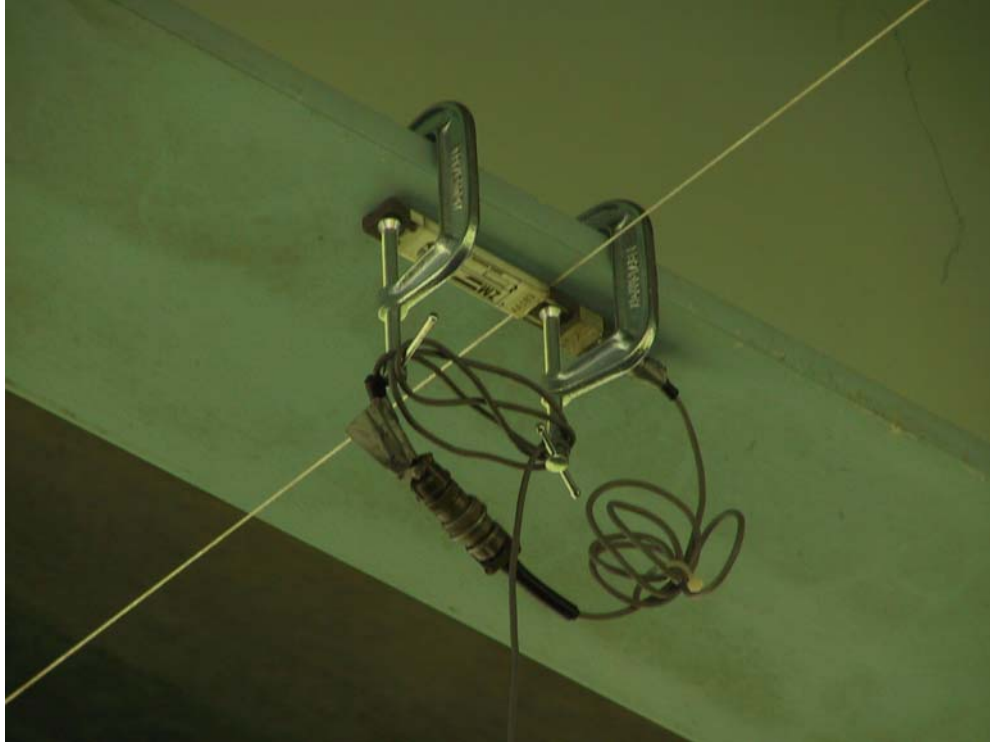
Figure 3.1 Removable Strain Transducer Mounted to the Lower Flange.
