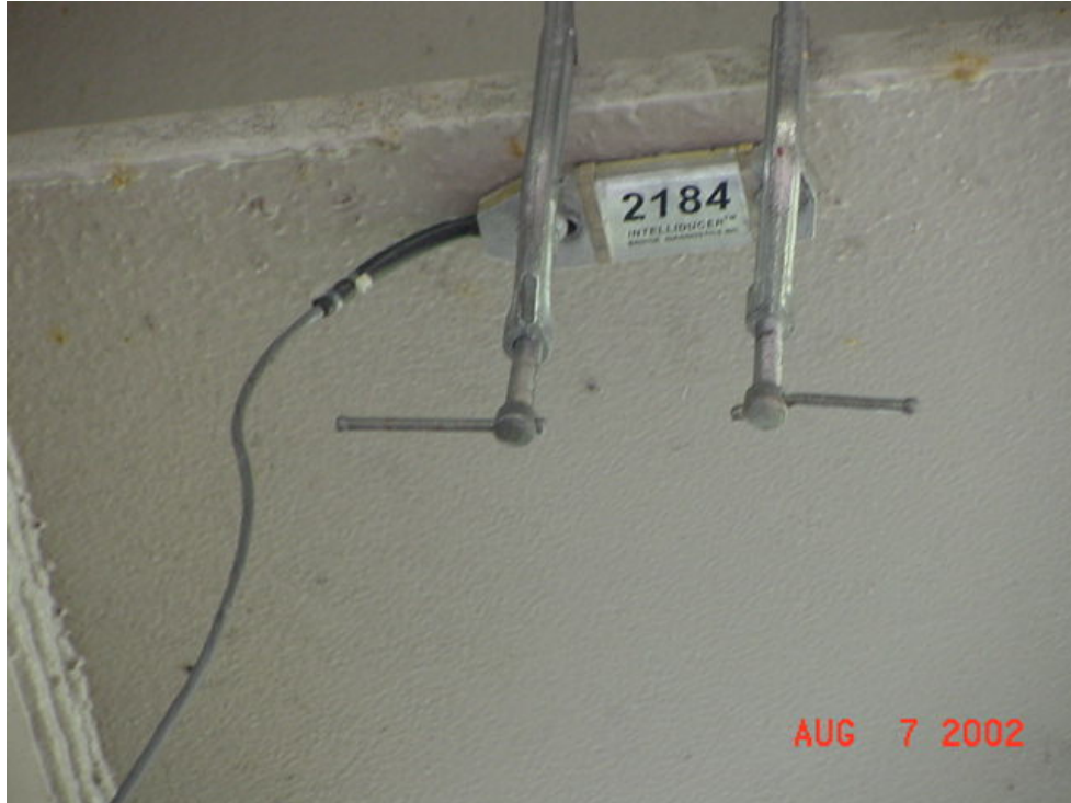
Figure 3.5 Installation of New Strain Transducer Purchased from Bridge Diagnostics, Inc.
