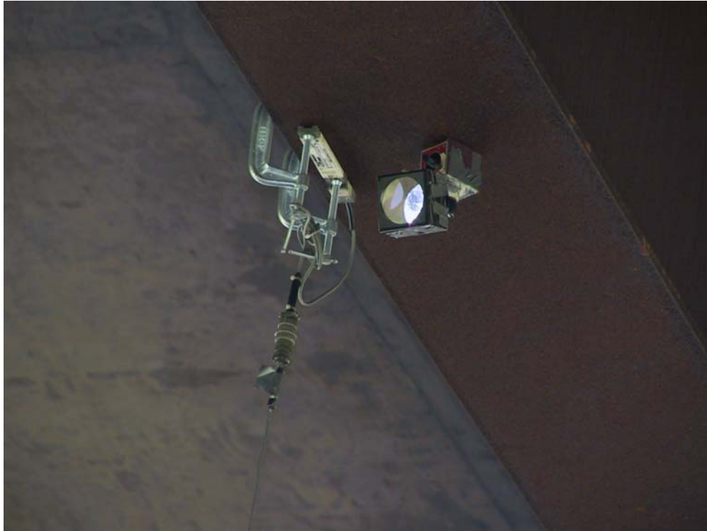
Figure 3.3 Prism Attached under Girder for Deflection Measurement
