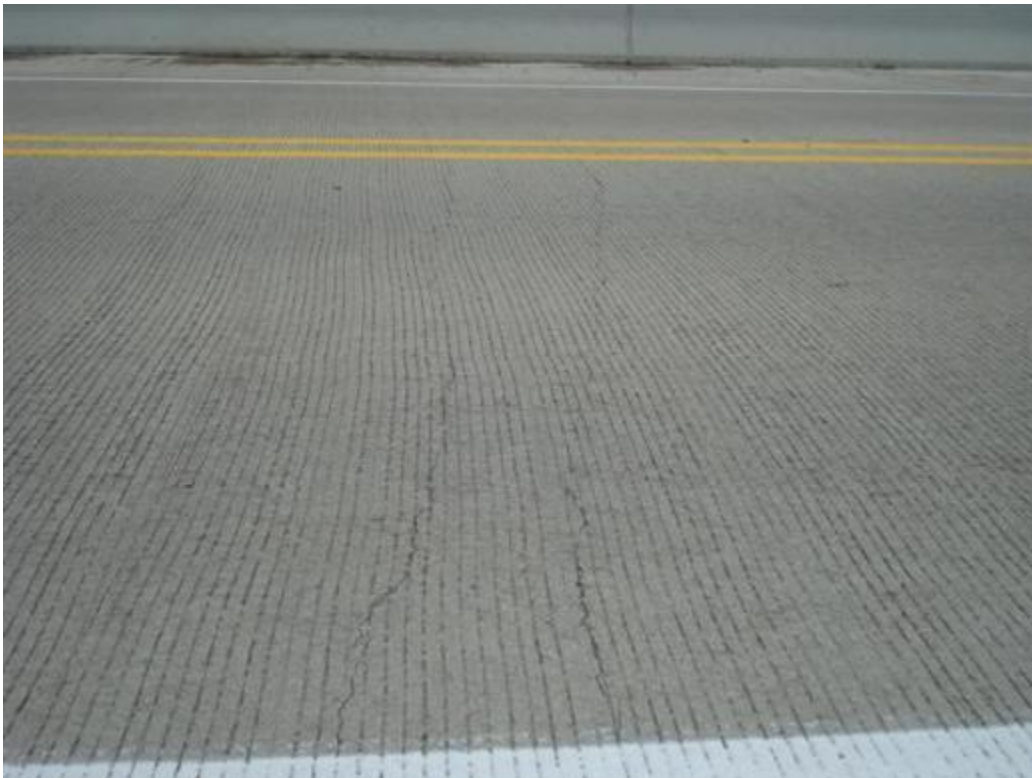
Figure 40. Bridge surface overall view (note longitudinal cracks)
