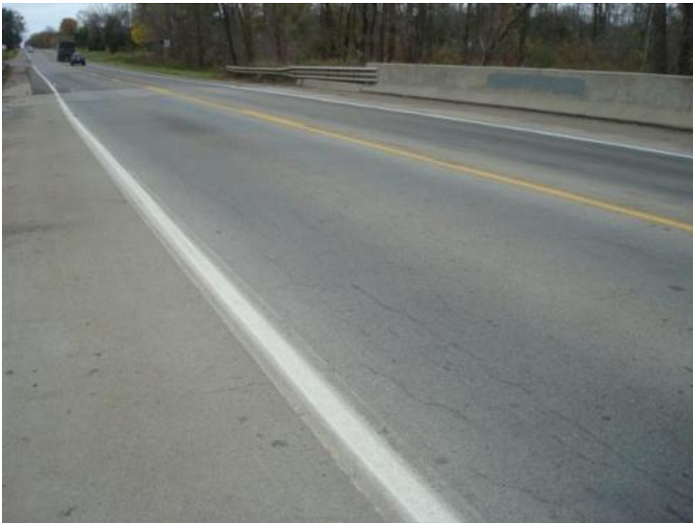
Figure 16. Longitudinal cracks
