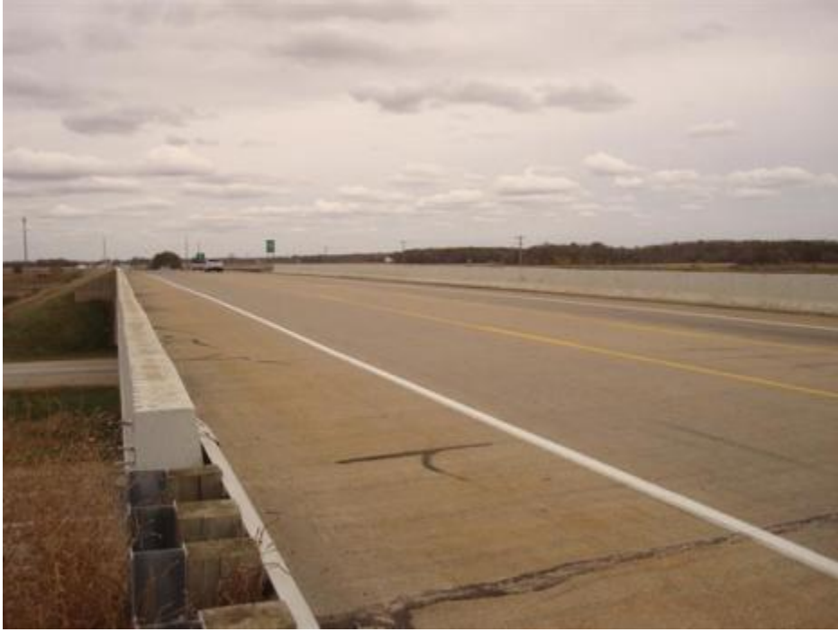
Figure 22. Overall bridge deck view
