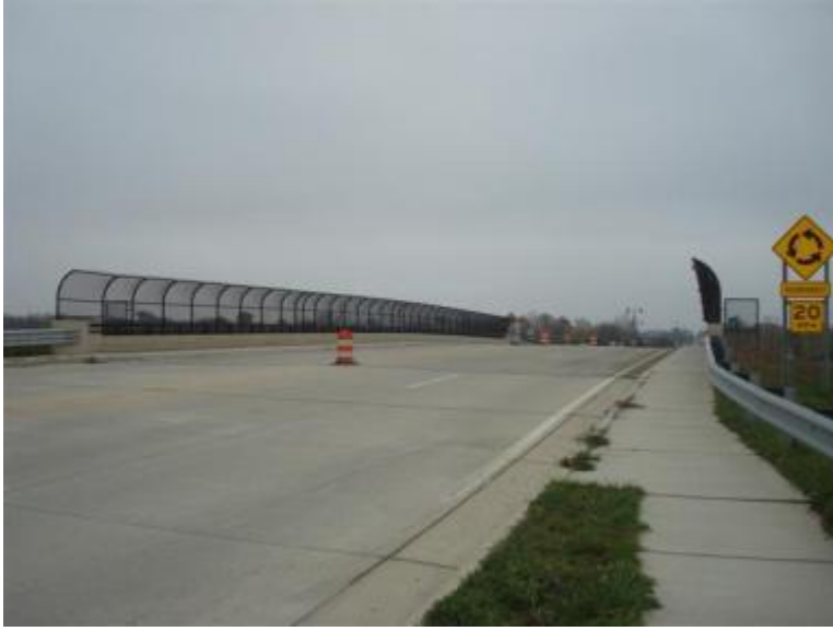
Figure 71. Bridge overall view
