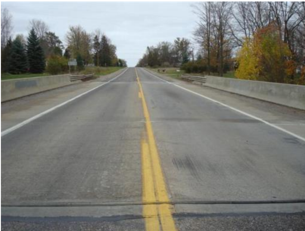
Figure 18. Deck overall vie
