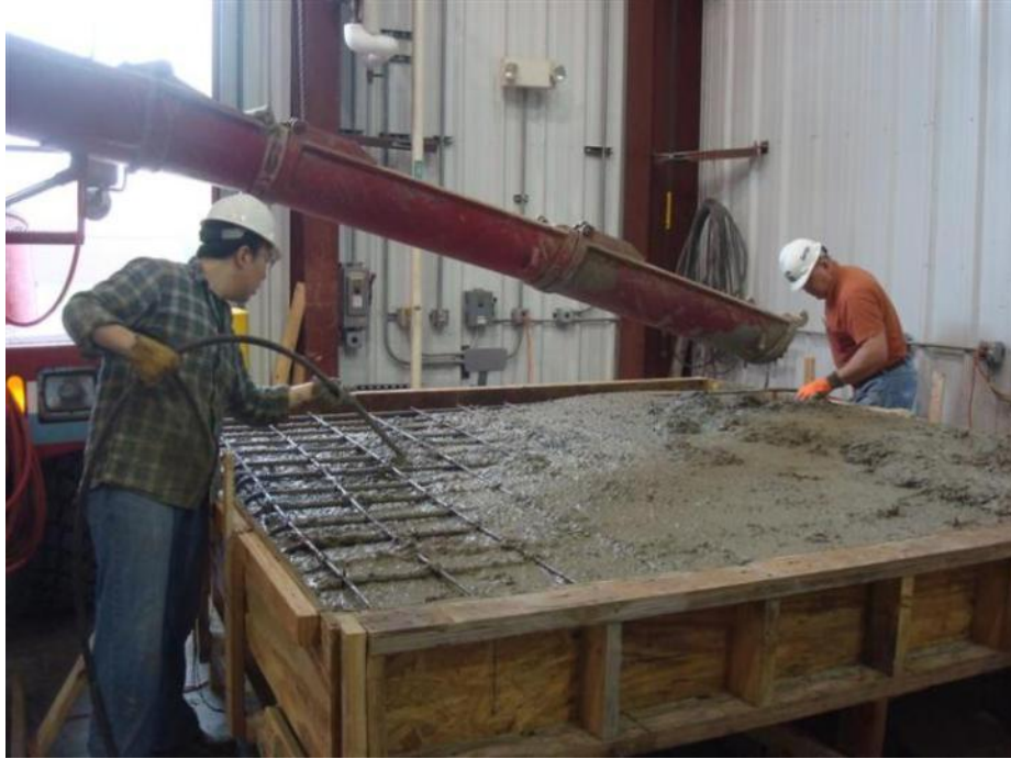
Figure 55. Placing and vibrating the concrete (test unit 3)
