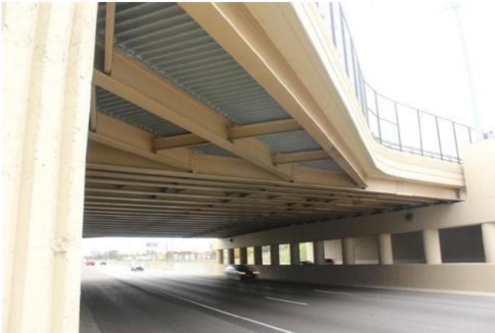
Figure 117. Bridge underside view
