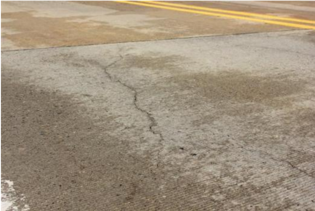
Figure 125. Longitudinal cracking
