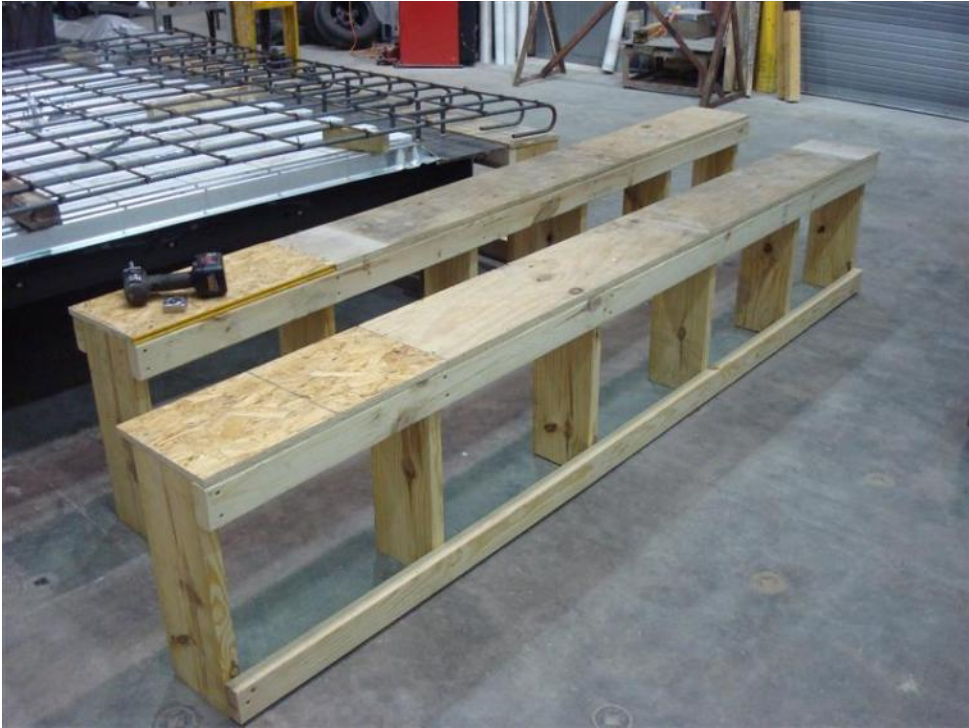
Figure 46. Cantilever forms bottom section
