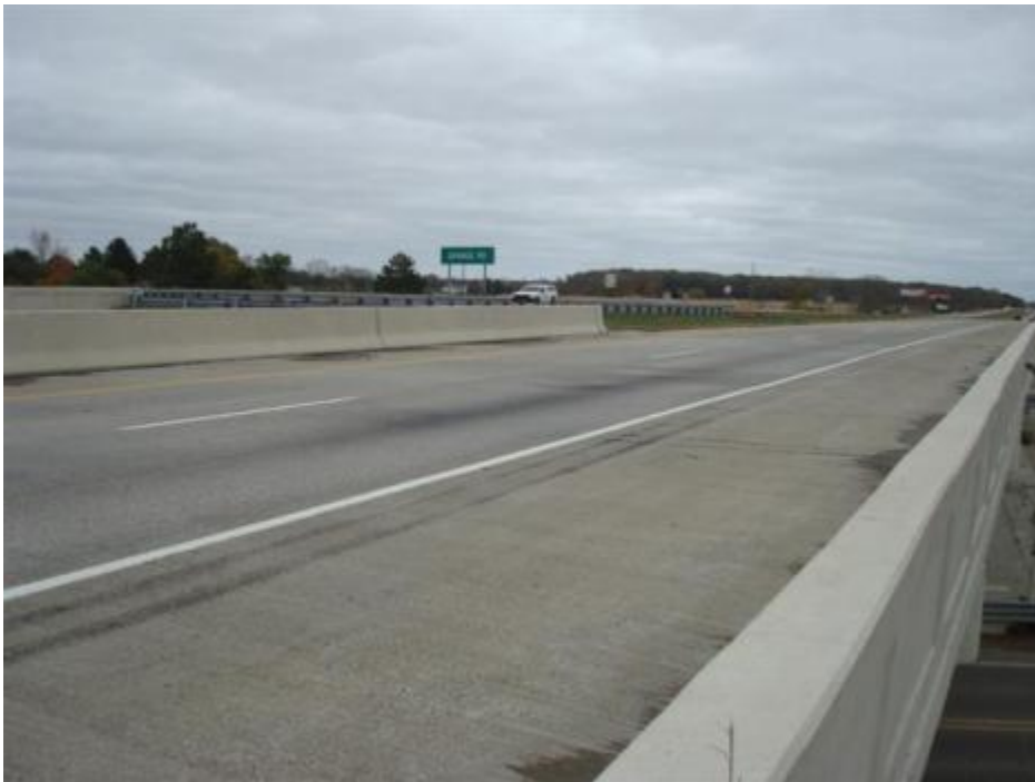
Figure 34. Bridge deck surface (other side)
