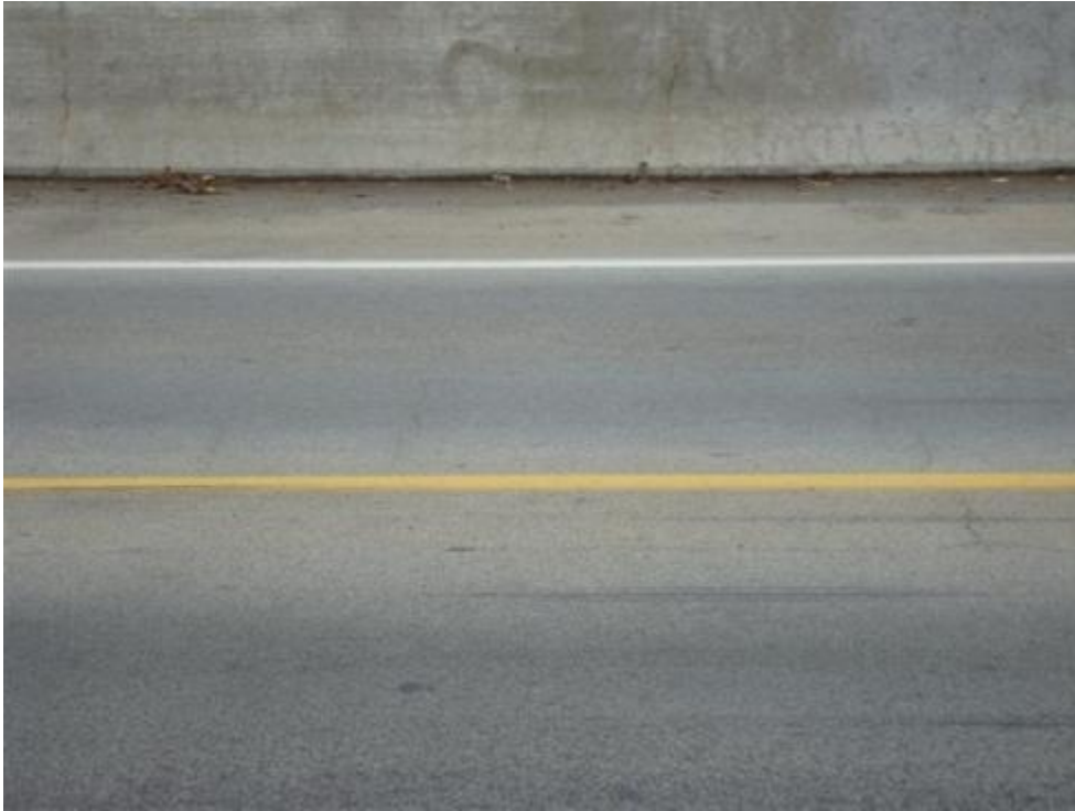
Figure 15. Transverse cracking in the deck
