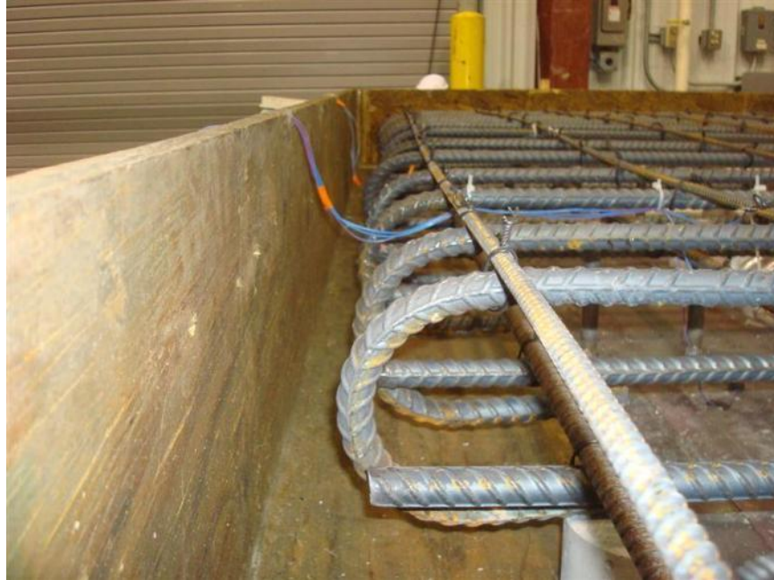
Figure 51. Reinforcing steel side cover (typical)
