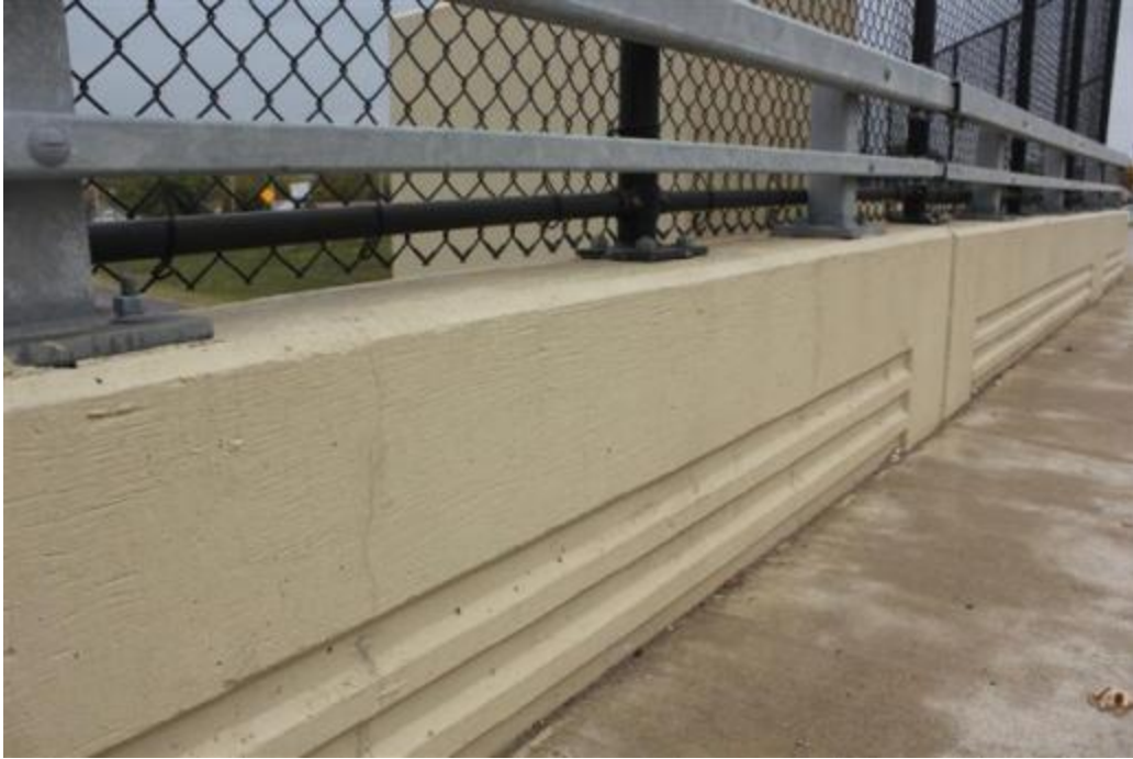
Figure 110. Cracking in barrier wall
