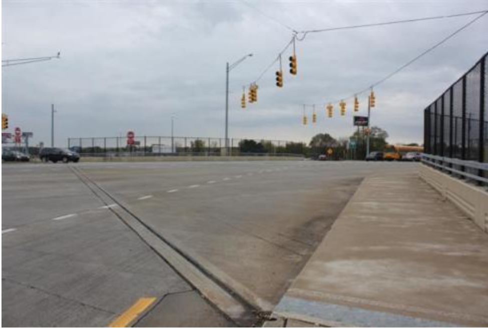
Figure 114. Bridge deck overall view
