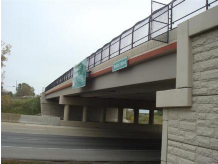
Figure 82. Overall bridge view
