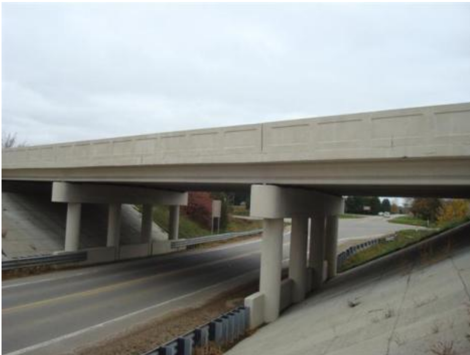
Figure 32. Overall bridge view
