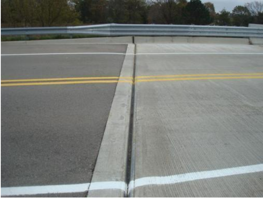
Figure 43. Bridge expansion joint (relatively clean of debris)
