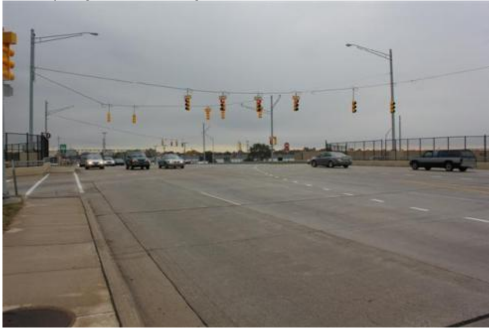
Figure 109. Bridge approach overall view
