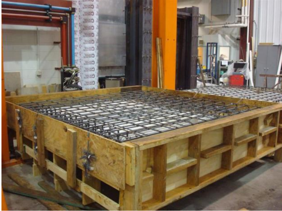
Figure 48. Completed formwork (all lumber forms are removable)
