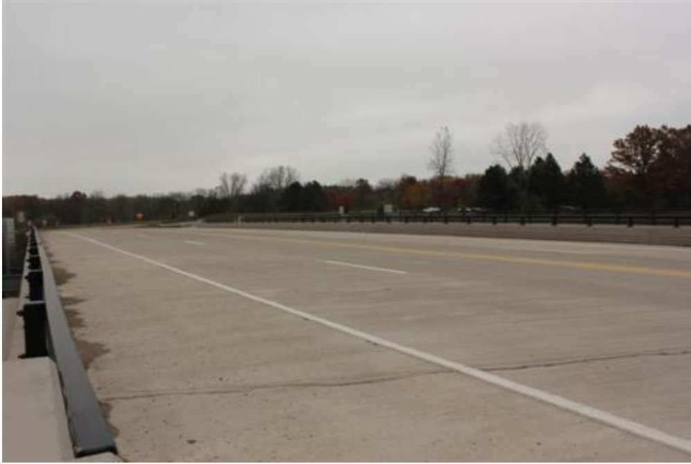
Figure 64. Bridge deck overall view
