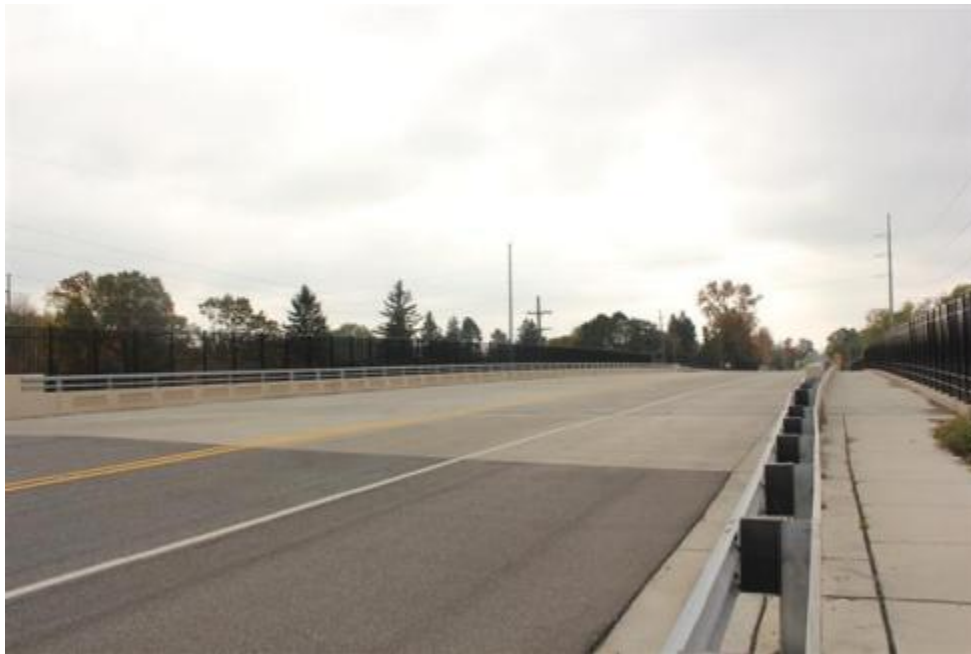
Figure 91. Bridge overall view
