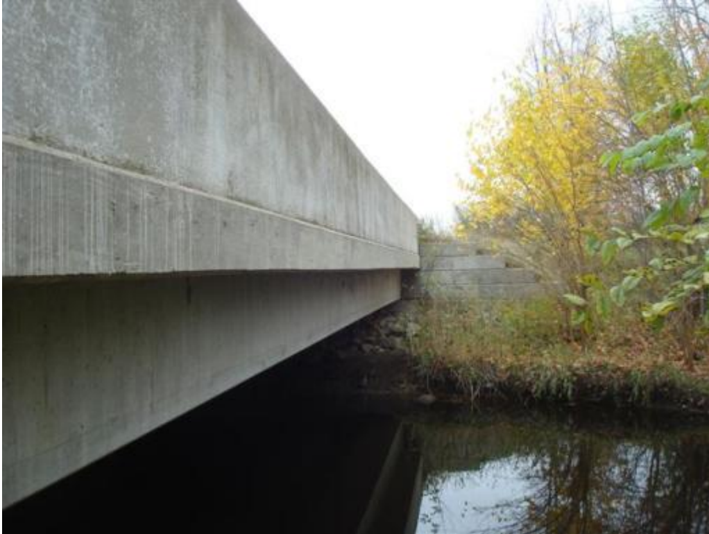
Figure 10. Bridge overall view
