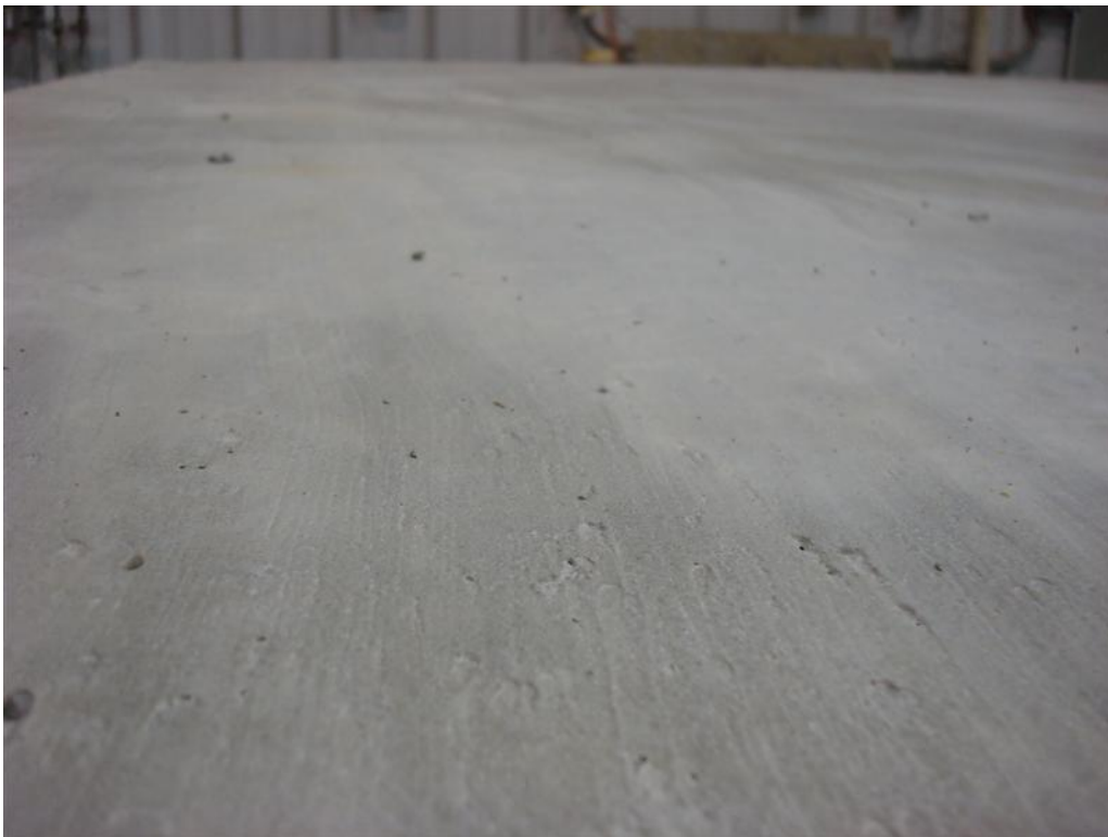
Figure 60. Close-up of completed test unit top surface (test unit 4)
