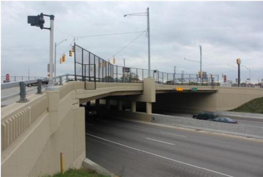
Figure 115. Bridge overall view
