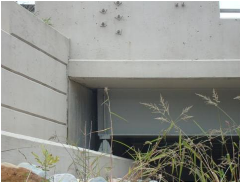
Figure 45. Semi-integral abutment detail
