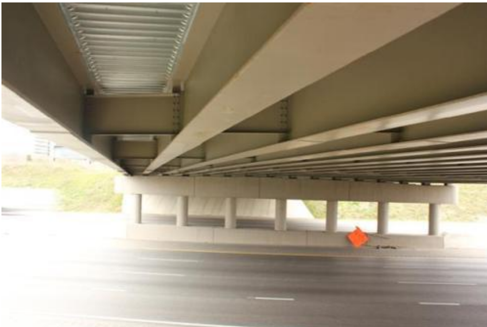
Figure 63. Bridge underside overall view
