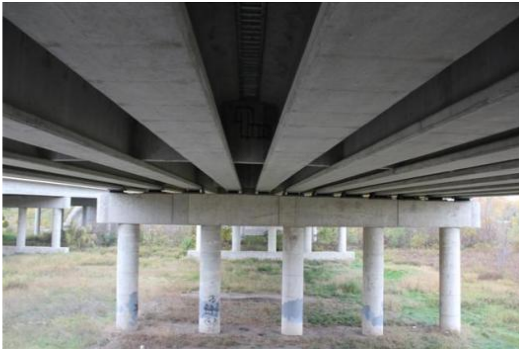
Figure 102. Bridge underside view (girder spacing is larger in the left side of the photo)
