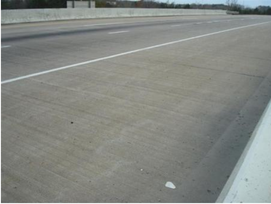
Figure 4. Overall deck view
