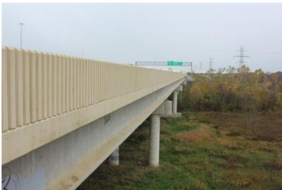
Figure 98. View of side of bridge
