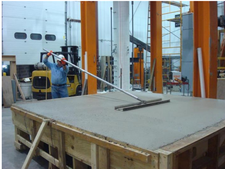
Figure 56. Bull floating the concrete surface (test unit 3)
