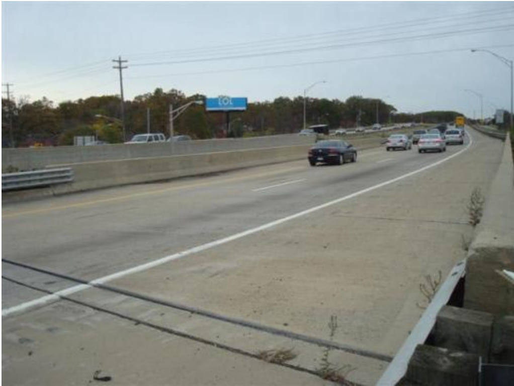
Figure 7. Overall bridge deck view
