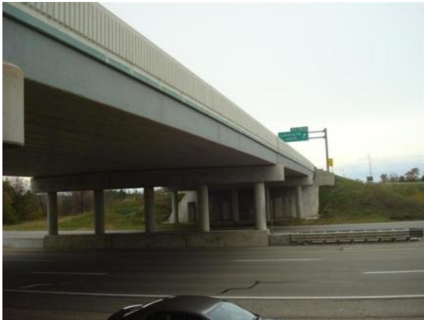
Figure 1. Overall Bridge View
