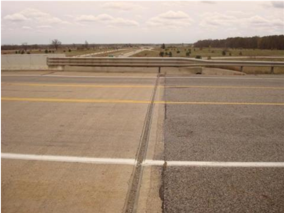
Figure 23. Bridge expansion joint and sleeper slab
