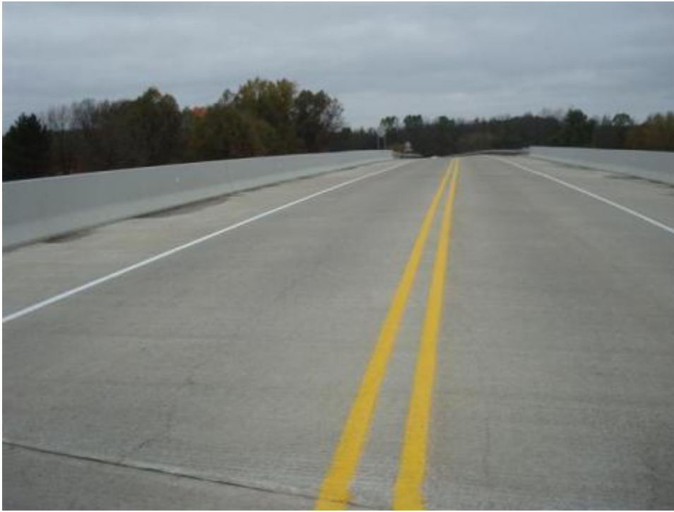
Figure 40. Bridge surface overall view (note longitudinal cracks)
