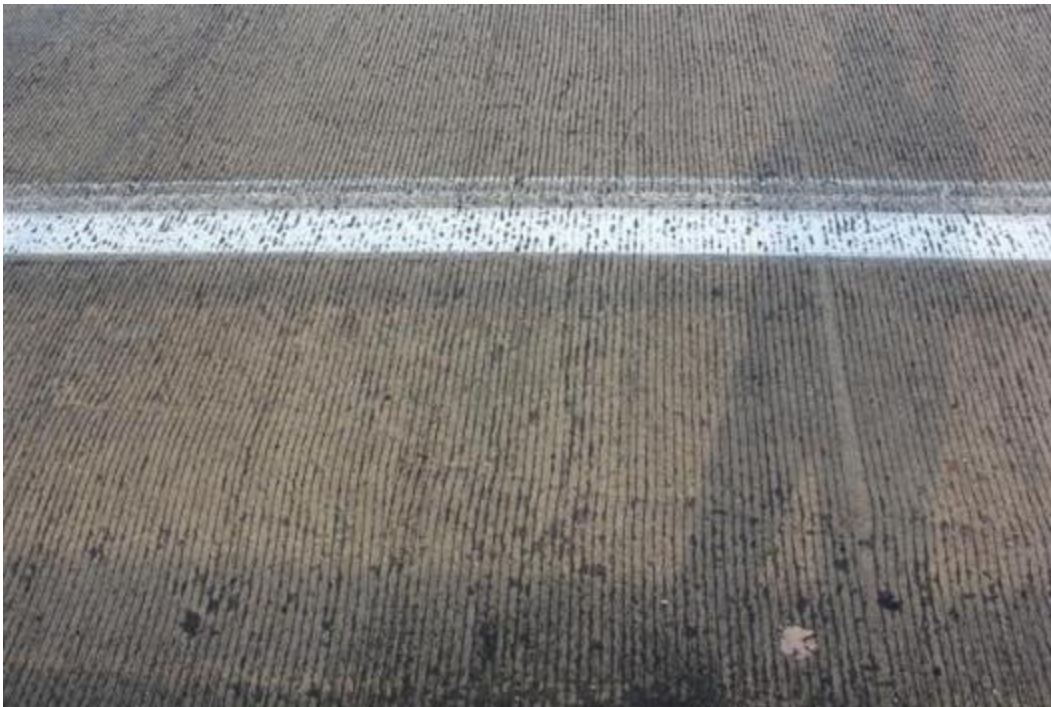
Figure 134. Transverse cracking
