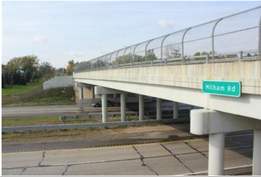
Figure 129. Bridge overall view
