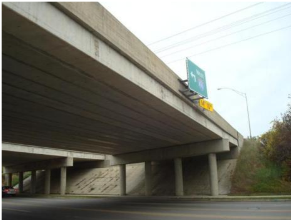
Figure 5. Overall Bridge View
