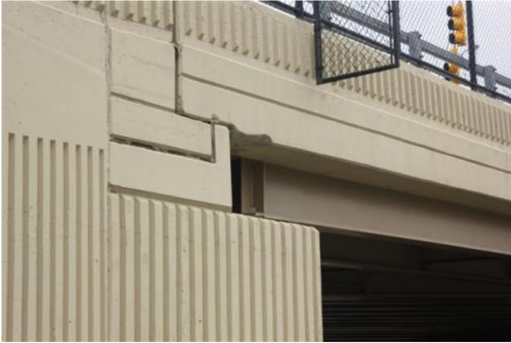
Figure 116. Non-integral beams/continuous deck at the abutment
