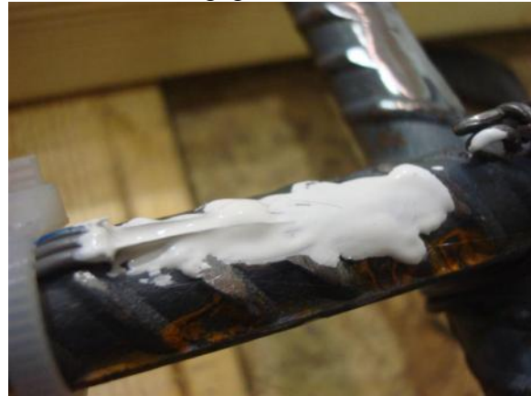
d) Assembly covered with M-Coat D
