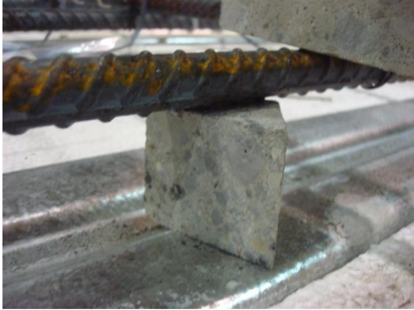
Figure 49. Concrete spacers for reinforcing steel (typical)
