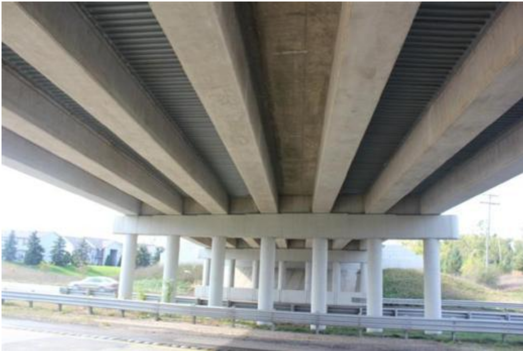
Figure 132. Bridge underside detail (note part-width construction area without SIP forms)
