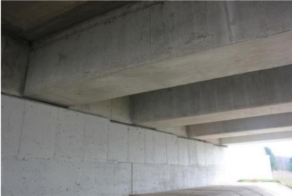
Figure 131. Abutment connection detail
