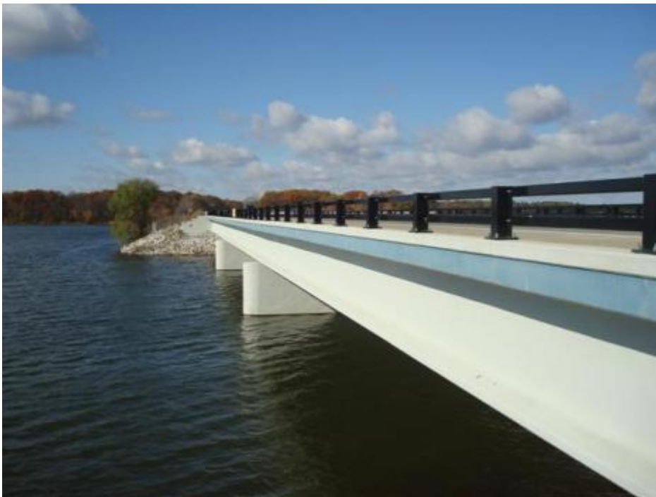
Figure 51. Overall Bridge View (Eastbound side)
