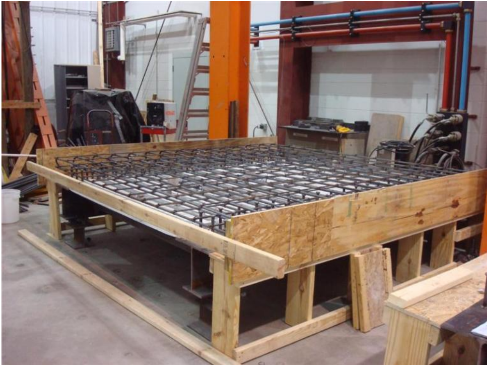
Figure 47. Completed cantilever forms
