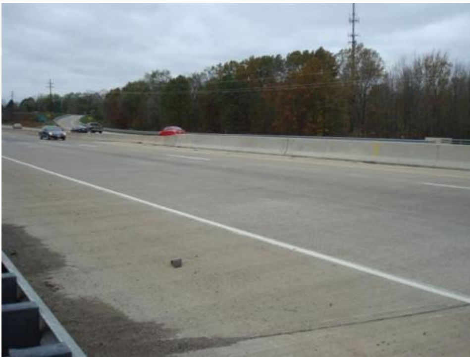
Figure 50. Bridge deck overall view
