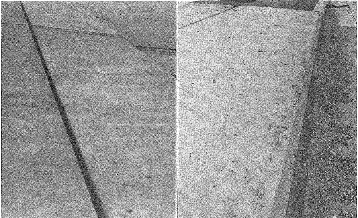
Figure 2. Typical scattered popouts on raised median.
