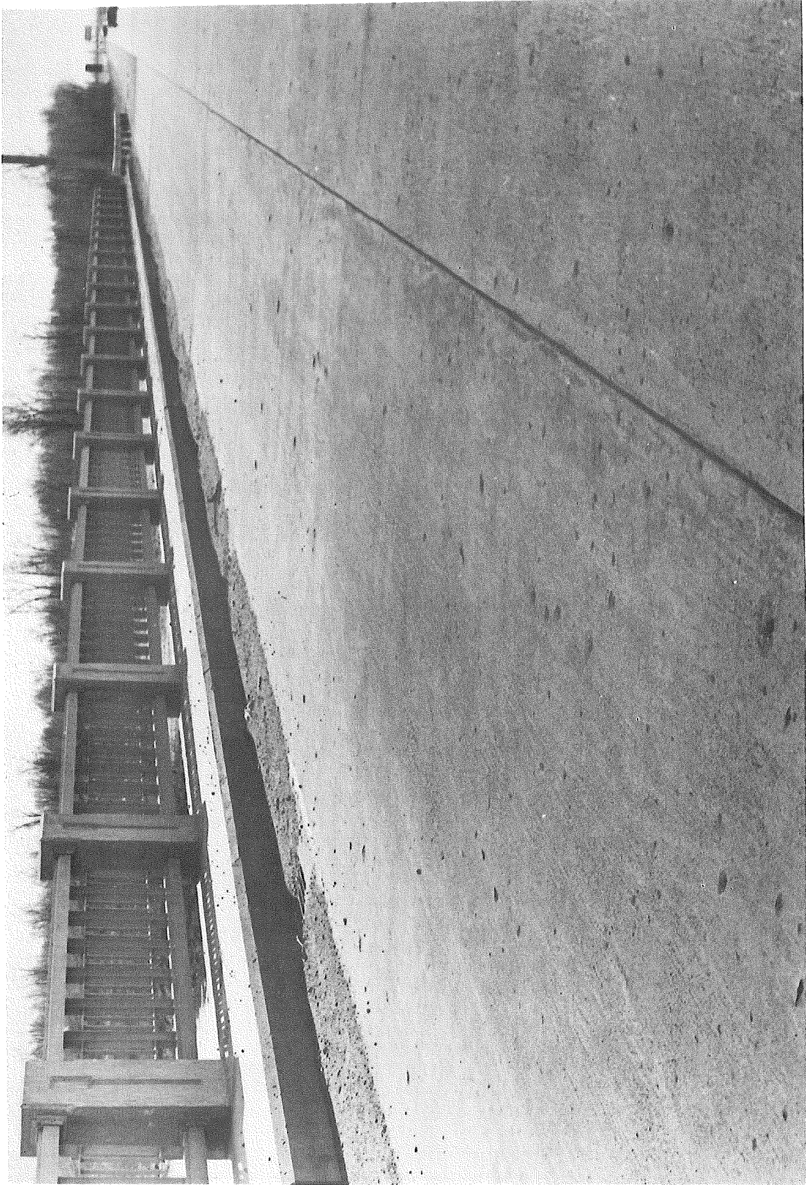
Figure 3. Looking south from bridge's easternmost lane, note alignment with shoulder on approach pavement, suggesting lighter traffic on this lane than the other six lanes. Incidence of popouts, however, is approximately the same.
