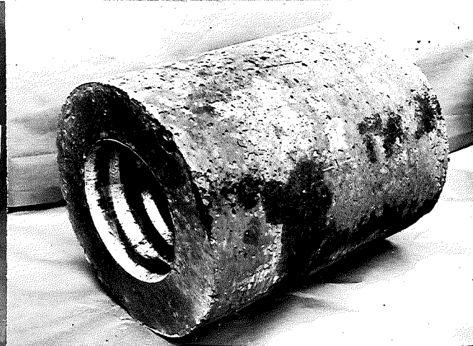
▲ TYPE 5. CORRUGATED STEEL CULVERT ENCASED IN A 5 INCH LAYER OF PLAIN CONCRETE.
