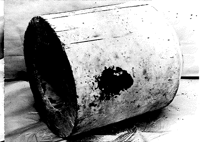
▲ TYPE 6. A PRECAST CONCRETE END SECTION WITH WALL THICKNESS OF 5 INCHES.
