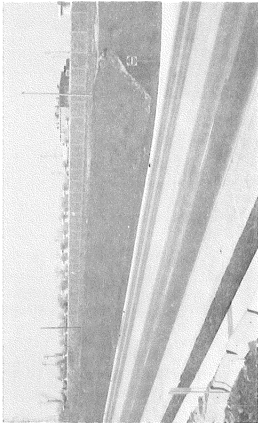
Enkamat stabilized slope shows no sign of failure despite water seepage.
