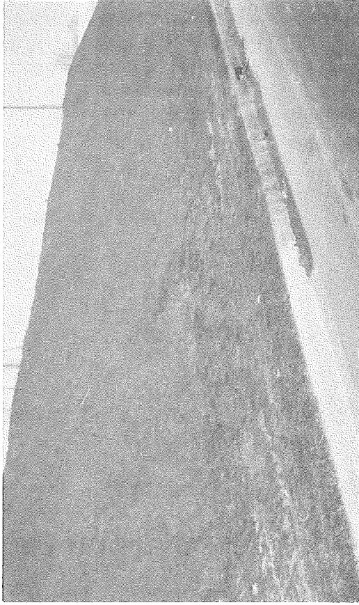
Enkamat stabilized slope shows no sign of failure despite water seepage.
