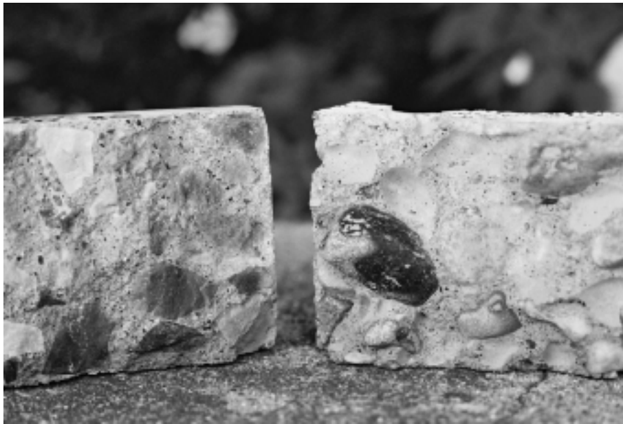
Figure 5.11 Crack roughness as observed from beam testing of concrete containing large size blend. Left: Rockwood (Pit # 58-8); right: Martin Aggrgate (Pit # 19-55).
