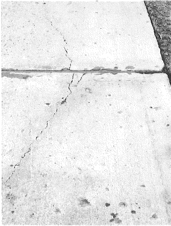
Sta 201+16, Proj 47-26, C6; constr 1949 (Nov '56)
