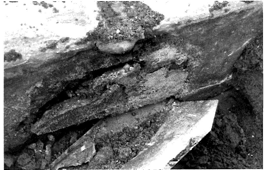
Sta 876+00, Proj 39-40, C4; constr 1953 (Apr '57)
