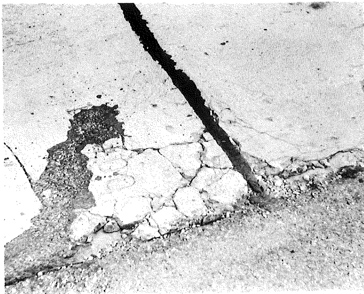
▲ Figure 3. Typical spalling at intersecting transverse and longitudinal joints. Sta 76+13; Proj 28-38, C2; constr 1948 (July '56)
