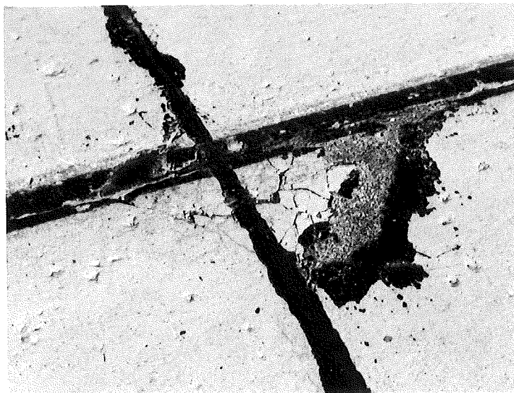
▲ Figure 3. Typical spalling at intersecting transverse and longitudinal joints. Sta 76+13; Proj 28-38, C2; constr 1948 (July '56)
