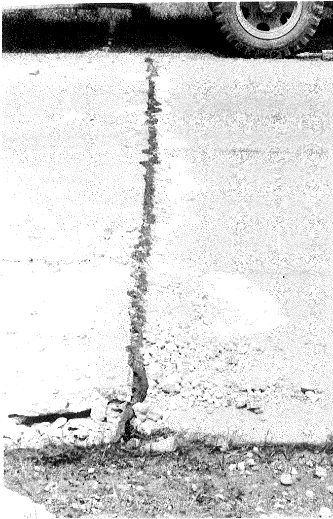
Figure 8. Joint failure in which dowel assembly device pushed upward, splitting the slab (left), with view after removal of overlying concrete (right). Proj 38-48, C5; constr 1952 (June '57).
