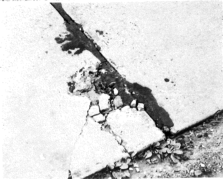
▲ Figure 4. Surface appearance of a pavement edge spall (top), with view of same joint after removal of spalled concrete (bottom). Sta 1016+83, Proj 39-40, C4; constr 1954 (Nov '54)
