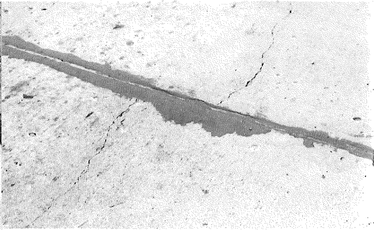
Sta 184+85, Proj 47-26, C6; constr 1948 (Nov '56)
