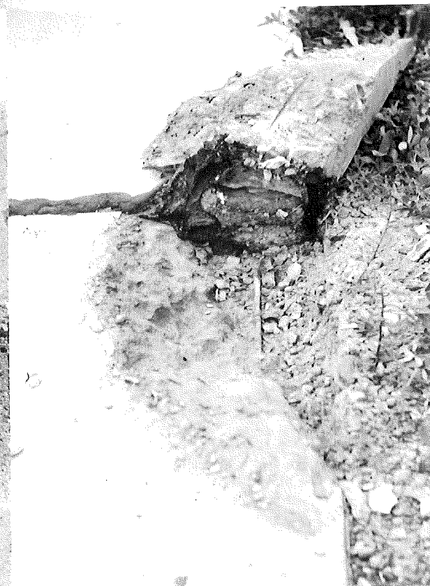
▲ Figure 4. Surface appearance of a pavement edge spall (top), with view of same joint after removal of spalled concrete (bottom). Sta 1016+83, Proj 39-40, C4; constr 1954 (Nov '54)
