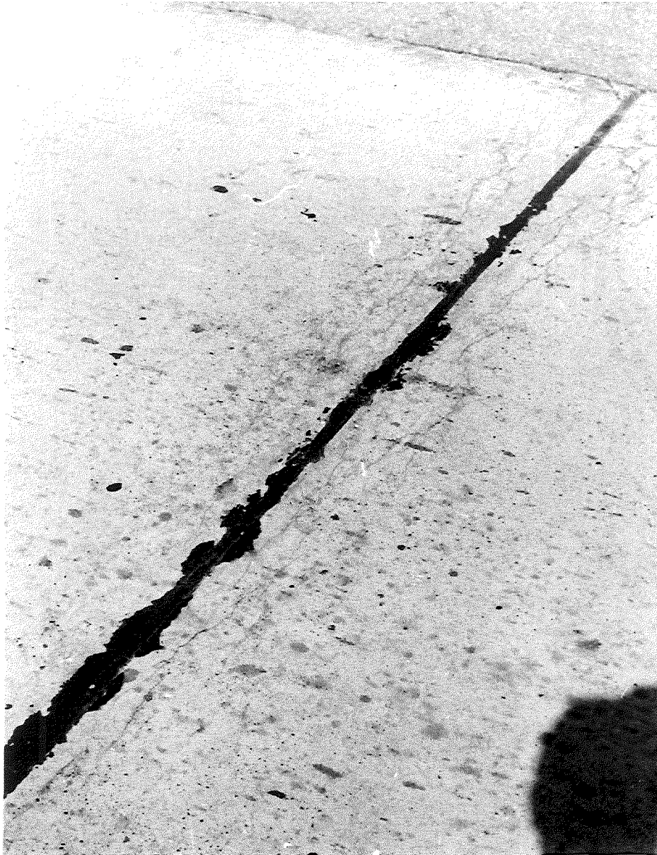
Proj 28-38; C2; constr 1948 (July '56) Sta 214+94
