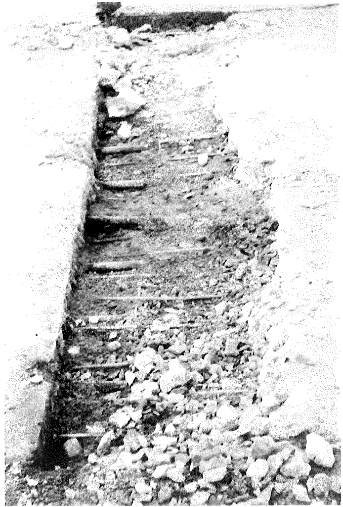
Figure 8. Joint failure in which dowel assembly device pushed upward, splitting the slab (left), with view after removal of overlying concrete (right). Proj 38-48, C5; constr 1952 (June '57).
