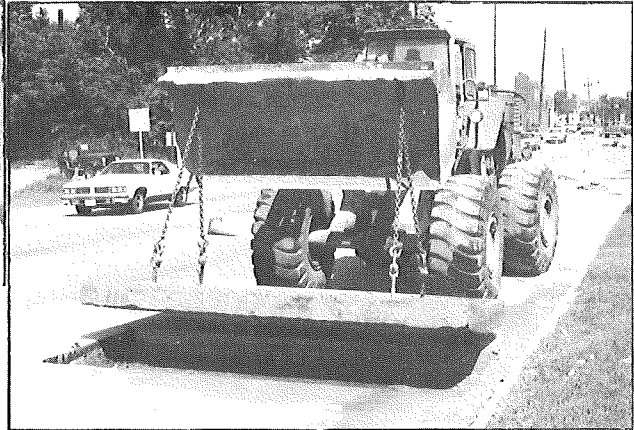
Figure 8b. The distressed concrete area is lifted out without disturbing the base. ▶
