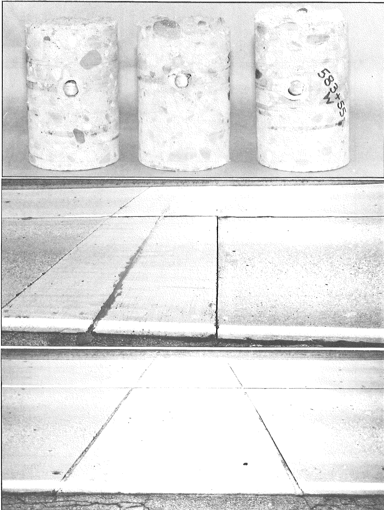
Figure 15. Failed tie bars caused by insufficient amount of grout around the bars (top), condition of repair with open and faulted tied joints after six years service (center), and condition of good performing six-year old dowelled repair (bottom); stage 3 repairs on I 94 in Jackson County, subjected to 3,500,000 ESALS.
