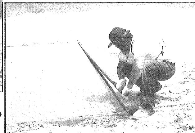
Figure 24b. Prior to the concrete gaining its initial set, the groove forming strips are removed. ▶
