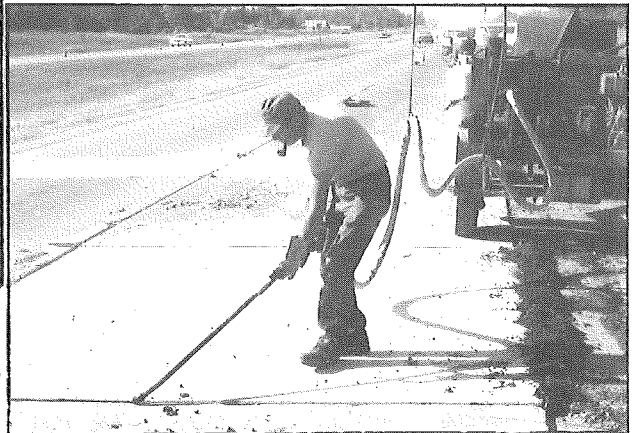
Figure 28b. A hot-poured rubber-asphalt sealant is installed in the joint grooves.
