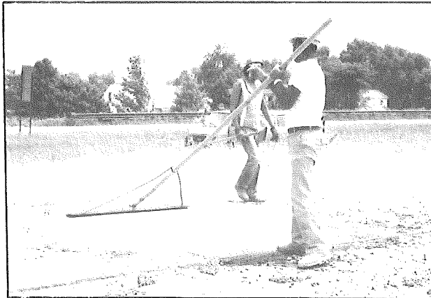
◀ Figure 21b. The surface of the concrete is finished by hand floating.
