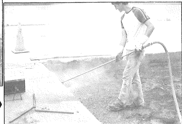
Figure 12b. Dowel holes are cleaned by using compressed air. ▶
