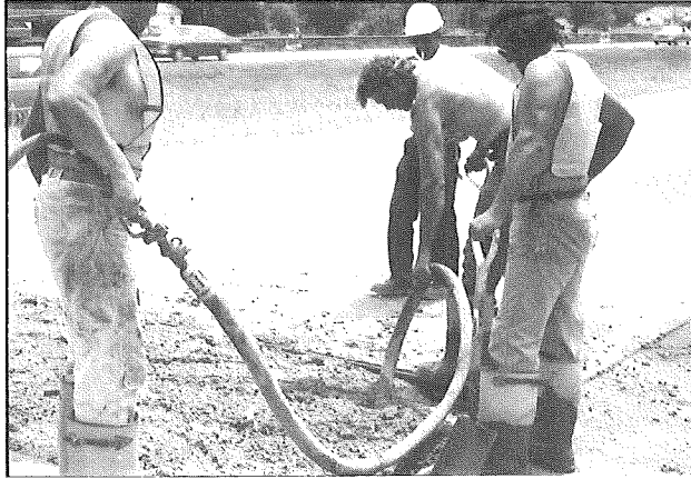
Figure 20b. The concrete must be struck-off using a vibrating screed. At least two passes must be made. ▶
