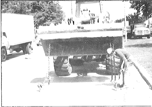
Figure 8b. The distressed concrete area is lifted out without disturbing the base. ▶
