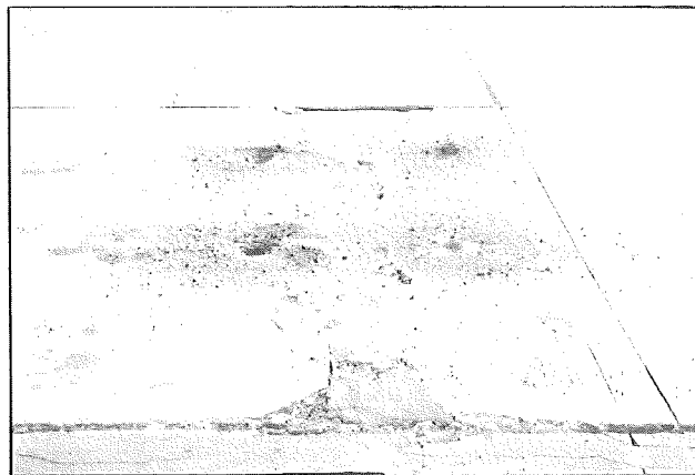
Figure 6b. The concrete between the double saw cuts has been removed to relieve compression in the slab. ▶
