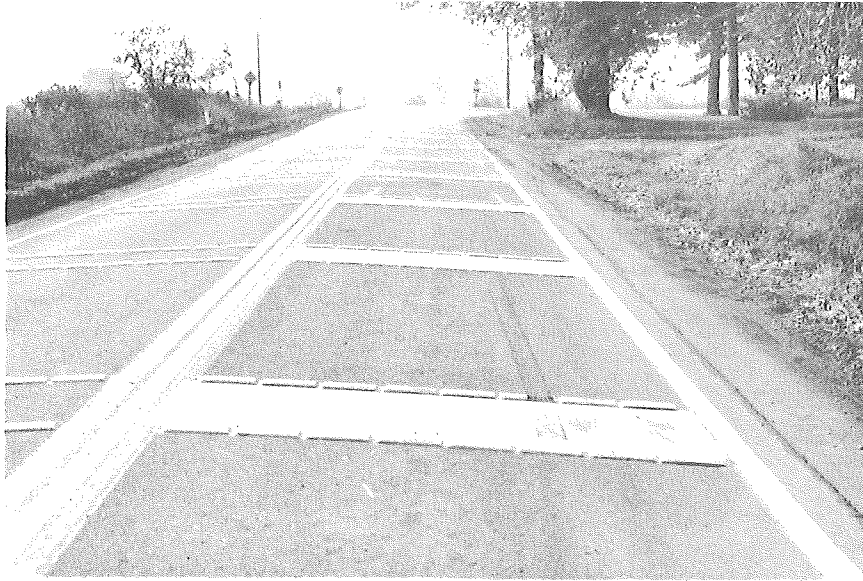
Fig. 13 - Rumble bars and paint stripes on M-106
