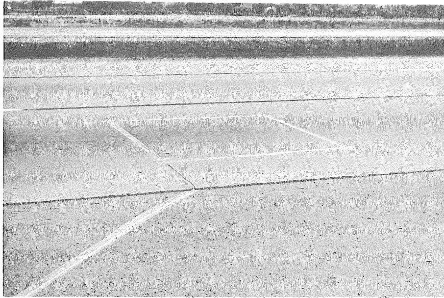
Fig. 5 - Induction loop taped onto pavement
