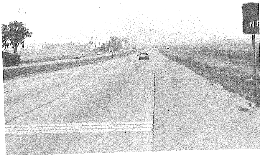
Fig. 4 - General appearance of transverse stripes on I-75
