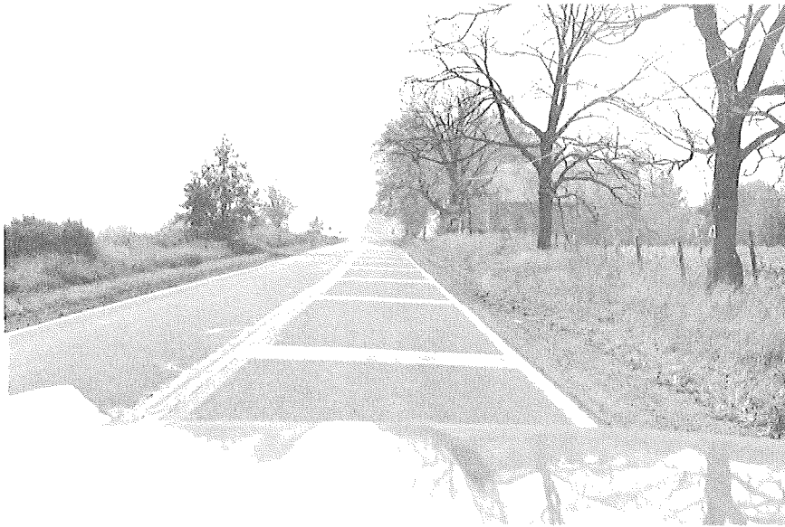
Fig. 11 - Paint stripes on M-106
