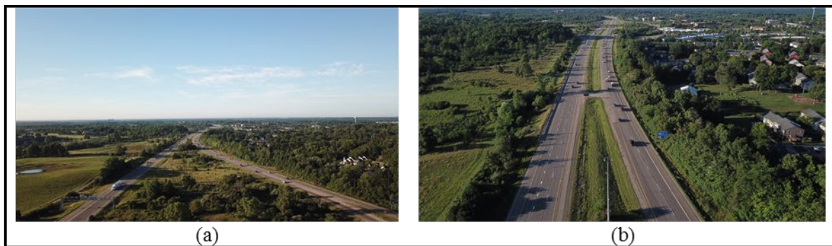
Figure 3.1.7: Screenshots of videos collected for the weaving area on July 31, 2020. (a) captures upstream. (b) captures downstream.
