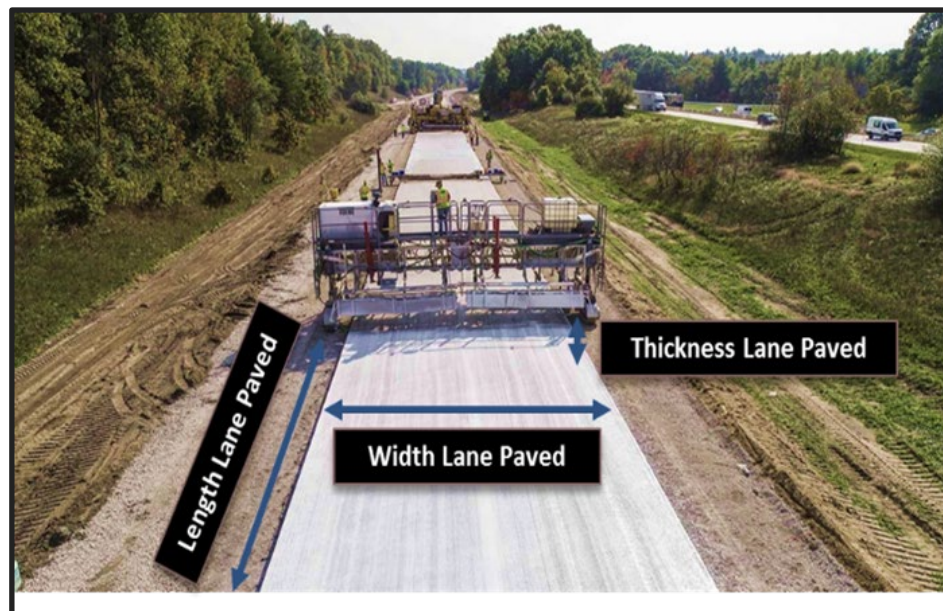
Figure 3.3.6: Example highway corridor geometric parameters (Photo from: https://www.bridgemi.com Photo Courtesy: MDOT).
