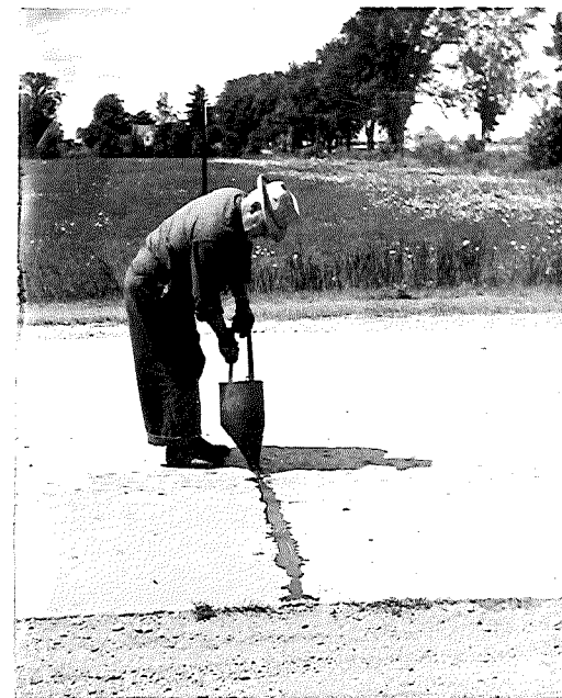
▲ FIGURE 4. RESEALING JOINT WITH HAND-POUR POT.
