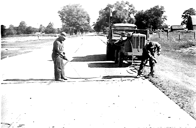
▲ FIGURE 2. RAKING AND AIR BLOWING OPERATION TO CLEAN JOINT FOR RESEALING.
