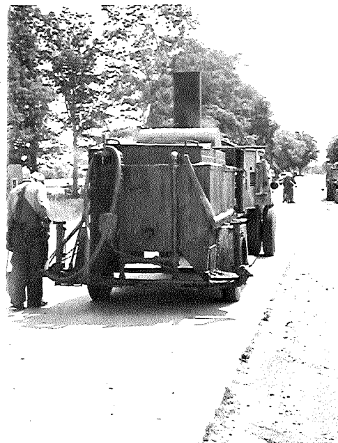
▲ FIGURE 3. DIRECTLY HEATED KETTLE FOR MELTING SEALING MATERIALS.
