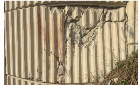
Deteriorated Panel
