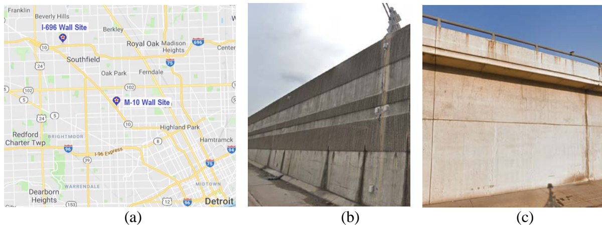
Figure 2.1. (a) Retaining wall site locations (Source: Google 2019); (b) I-696 Wall
