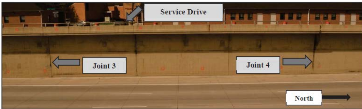
Figure 1.11. Retaining wall on M-10 (from Cerminaro 2014)
