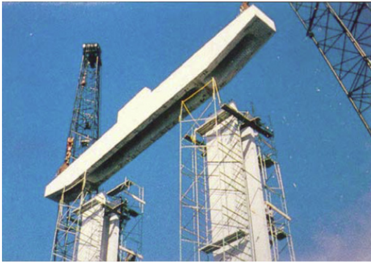
(e) Inverted-U section bent cap (Source: Culmo 2009)
