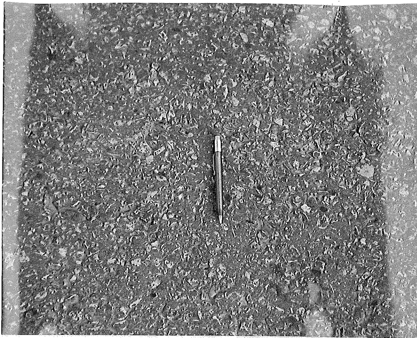
Figure 2. Dolose & Shepard Aggregate in Resurfacing 1 mile east of Three Oaks on M-60 .
