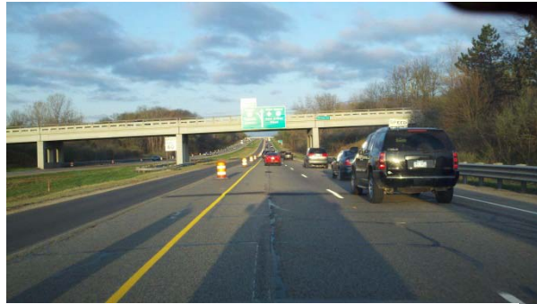
Figure 2 - New Construction on M-14
