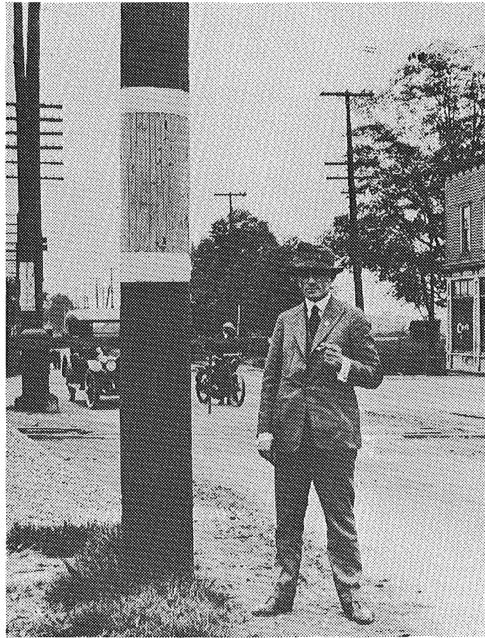
WHEN TELEPHONE POLES MARKED THE WAY-- Credit for developing the first systematic road-marking system in the U.S. goes to William B. Bachman (above) of Detroit, who in 1912 began marking roadside telephone poles in different colors to designate different routes. By 1920 he had banded 2,000 miles of Michigan highway poles, the forerunner of a national system of uniform signing that came into existence in 1927.
