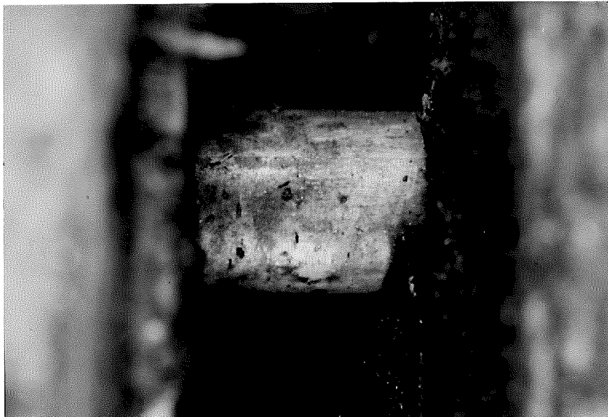
Figure 2. Surface condition typical of Monel and stainless steel sleeved dowels. Brown stains do not indicate corrosion.
