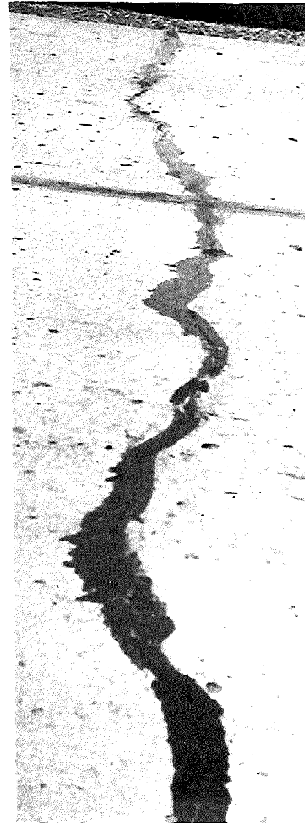
A. OVERALL VIEW
