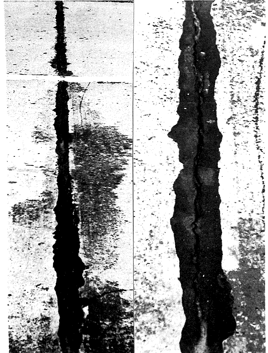
A. OVERALL VIEW
