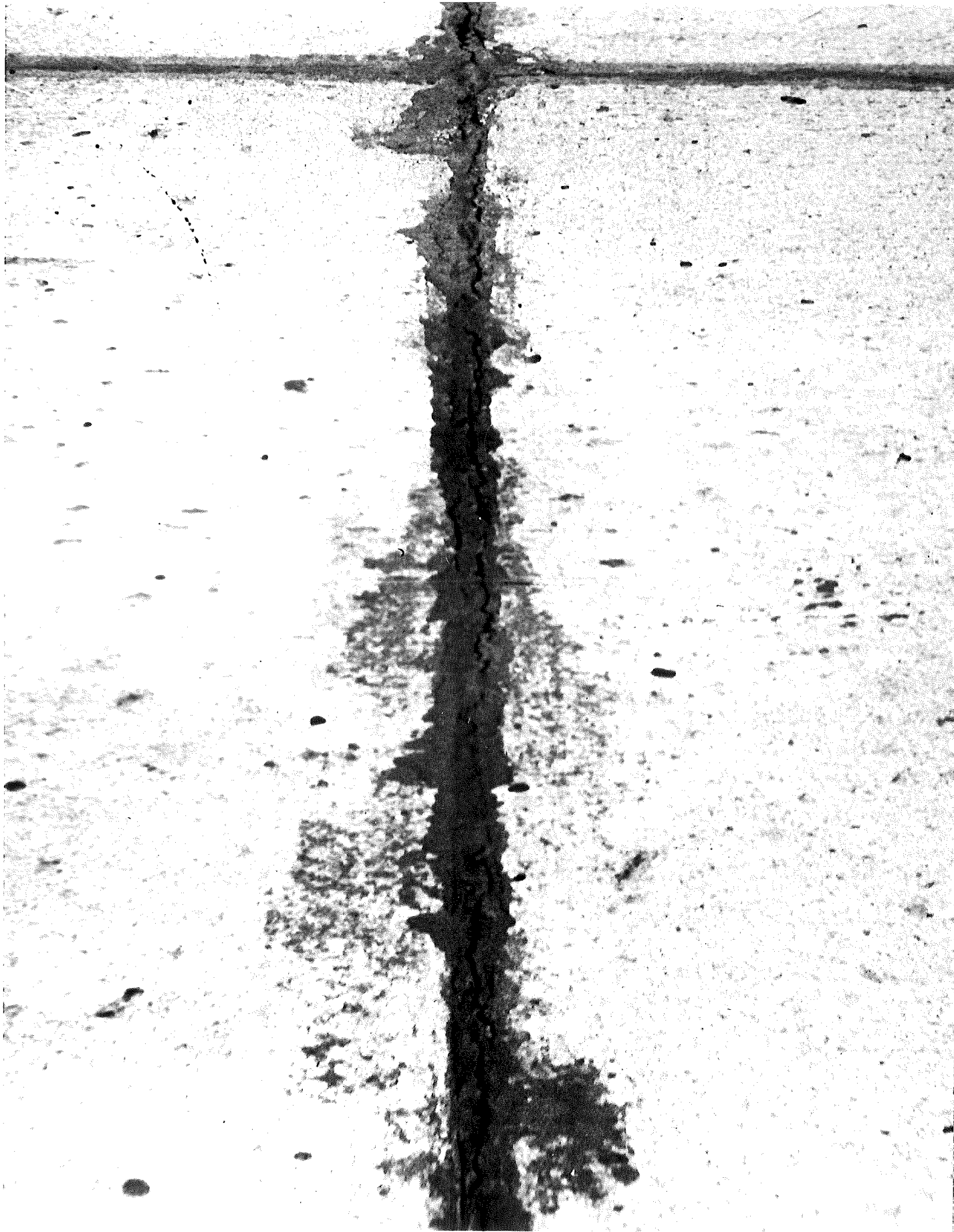
▲ FIGURE 8. STA. 280+32 EXPANSION JOINT RESEALED WITH BRAND D SEALER.
