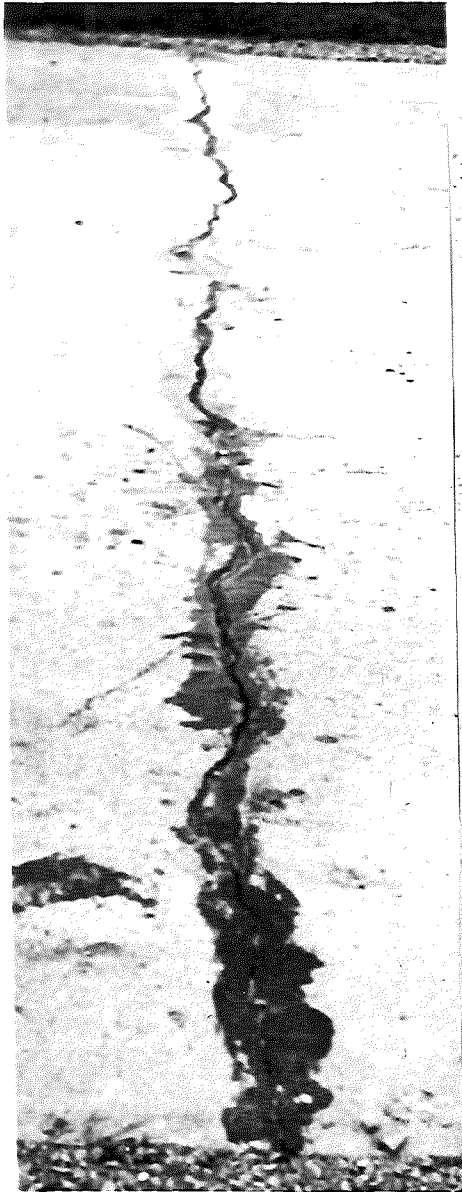
A. OVERALL VIEW
