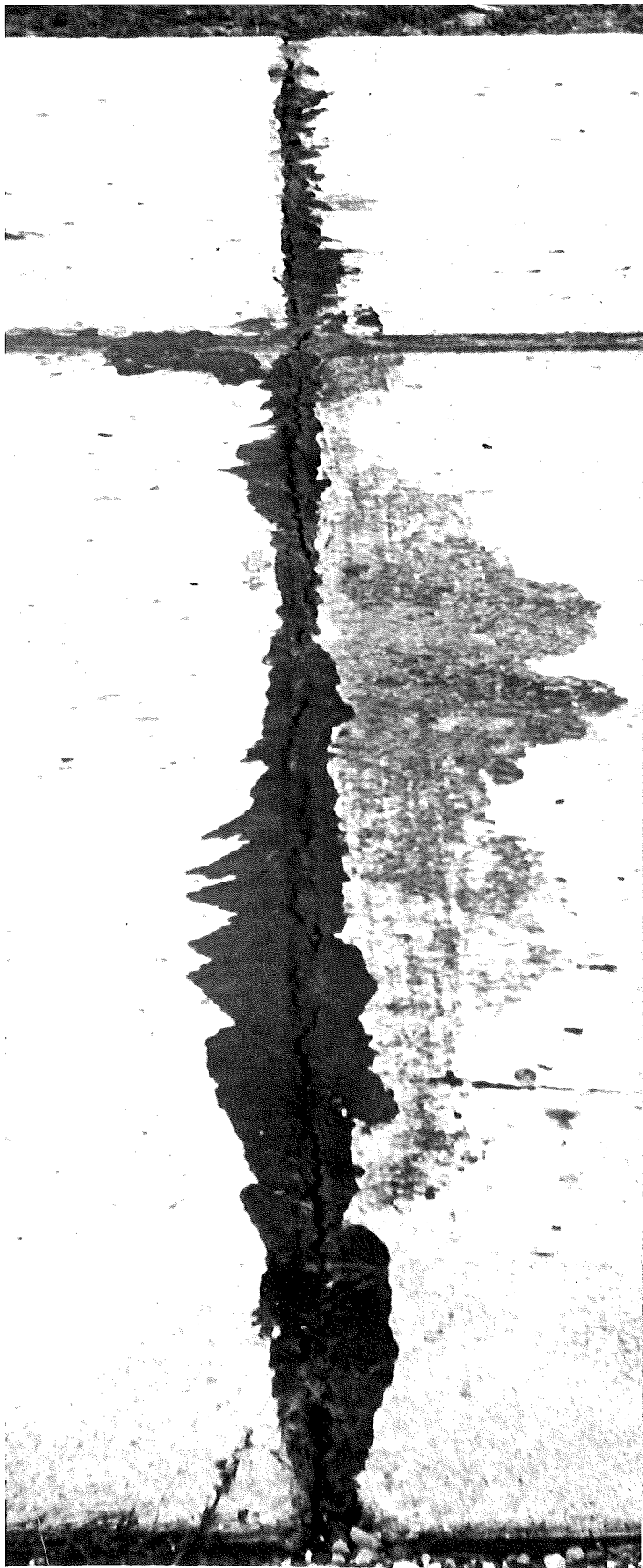
A. OVERALL VIEW
