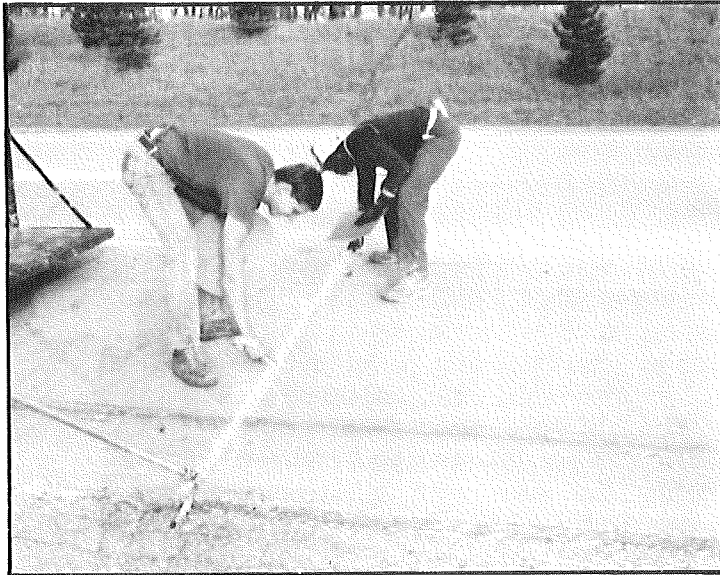
Figure 10. Installing and tooling silicone sealant.
