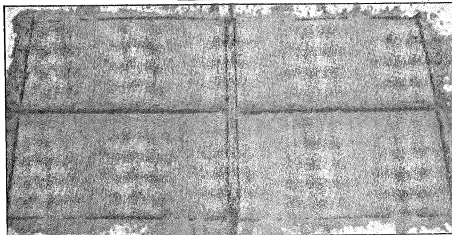
Figure 8. Finished repair before sealing joints.
