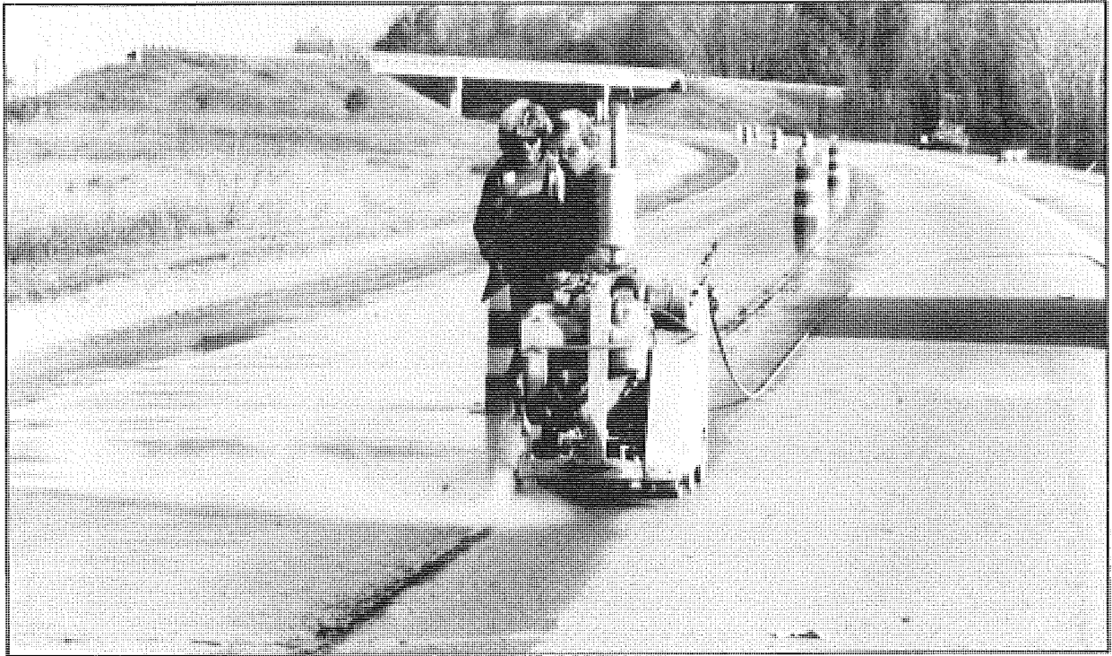
Figure 12. Resawing longitudinal joint groove.
