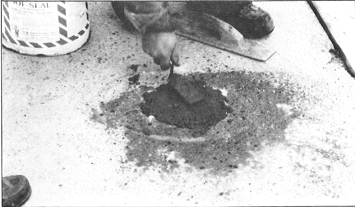
Figure 17. Placing fast-set mortar in pop-out.
