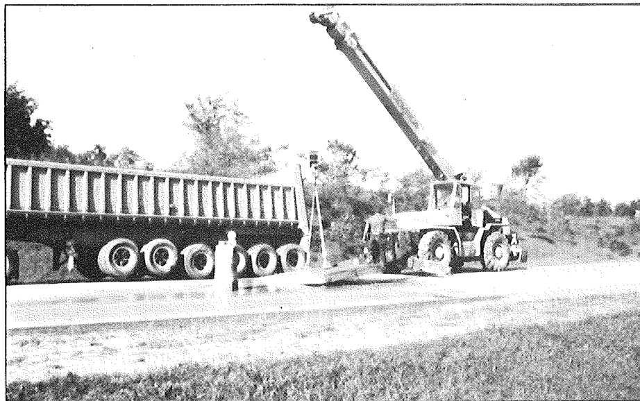
◀ Figure 1. Removing distressed pavement section.
