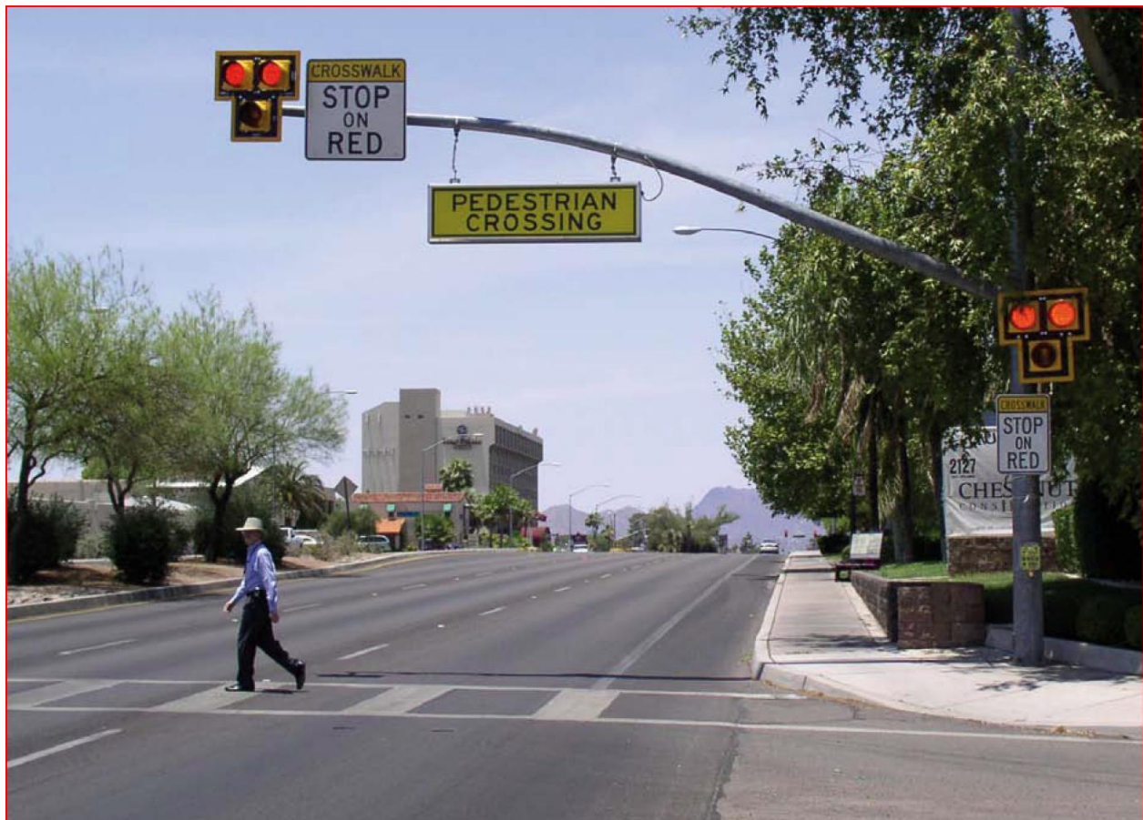
Figure 14. A HAWK pedestrian intersection (Source: FHWA, 2010)
