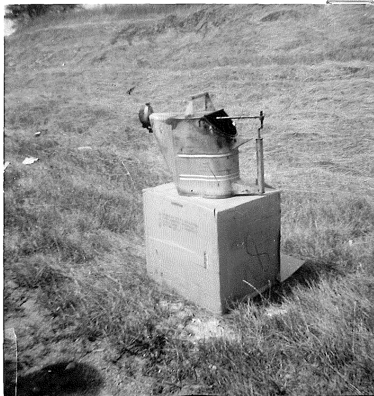
5. Pouring Pot US-16 near Lan- sing airport. BRD--8-18-47
