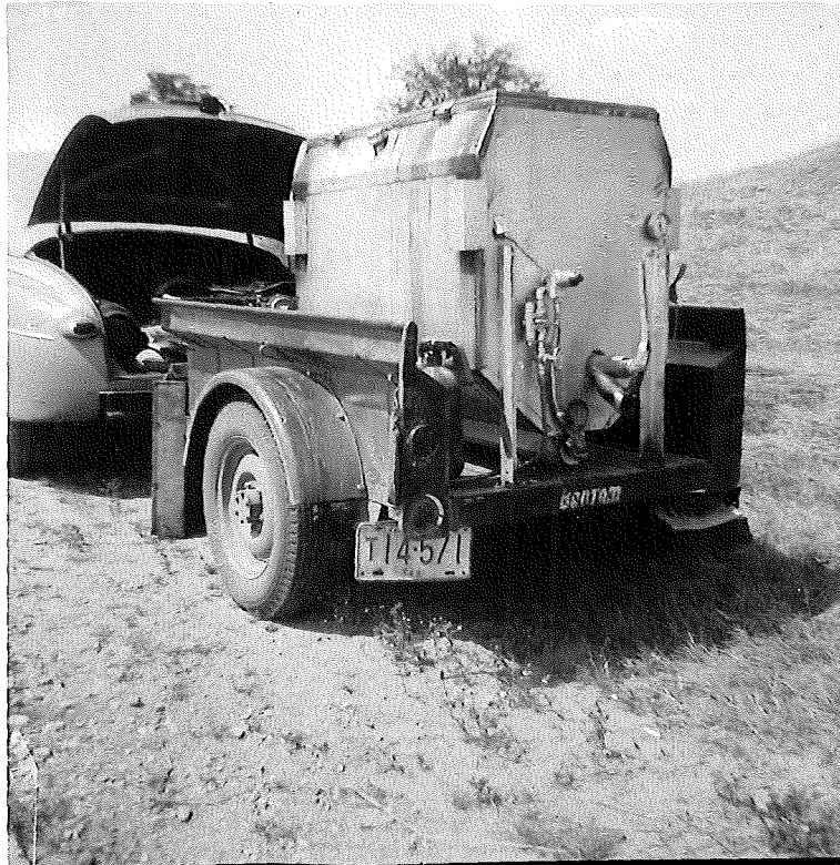
3. Rear view of heater. US-16 near Lansing airport. BRD--8-18-47
