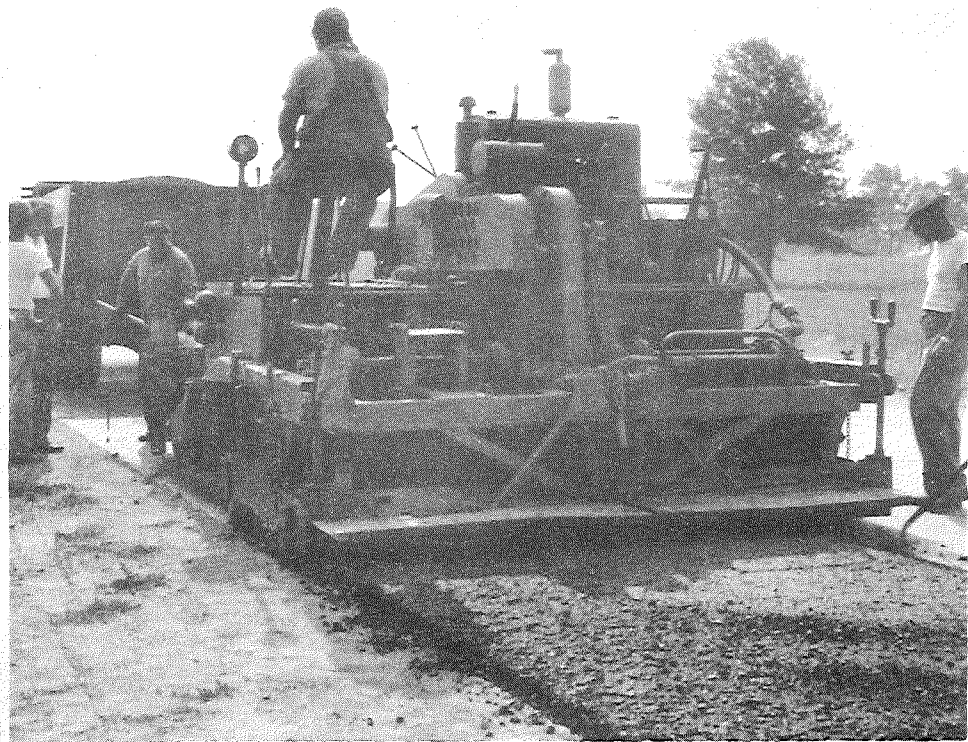
Spreader placing 8-ft binder course over reinforcing sheet.
