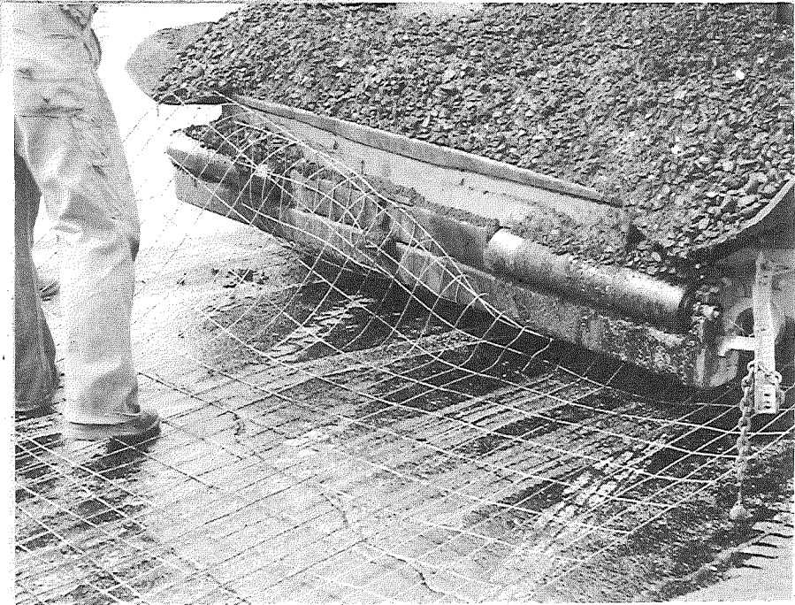
▲ Figure 6. "Hold-down device" used to depress reinforcing sheets under paver.
