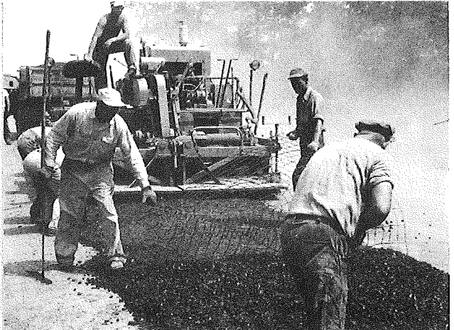
Removal of full width of buckled sheet from binder course.
