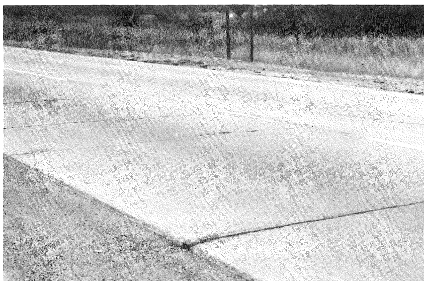
Figure 1. Typical appearance of original 1943 concrete pavement in July 1955.
