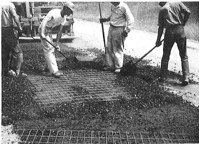
Installing new full width sheet to replace buckled steel, and replacing bituminous concrete by hand.
