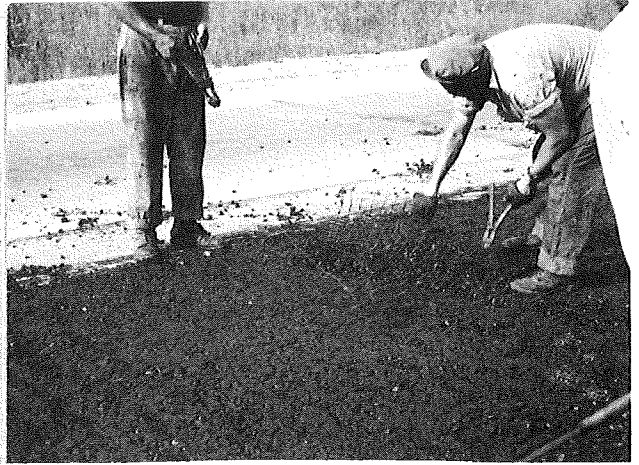
Smaller area of buckled steel.
