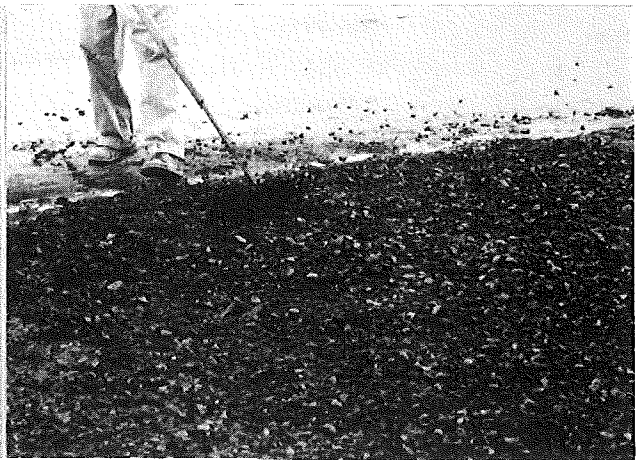
Installing new full width sheet to replace buckled steel, and replacing bituminous concrete by hand.
