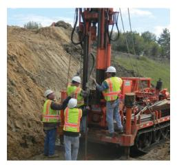
Researchers installed sensors by pushing them into the ground with a common drill rig.
