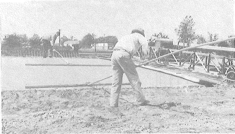
▲ Figure 19. After Partial Smoothing by the Second Spreader, the Finisher-Float Combination Completes the Mechanical Finishing of the Concrete.
