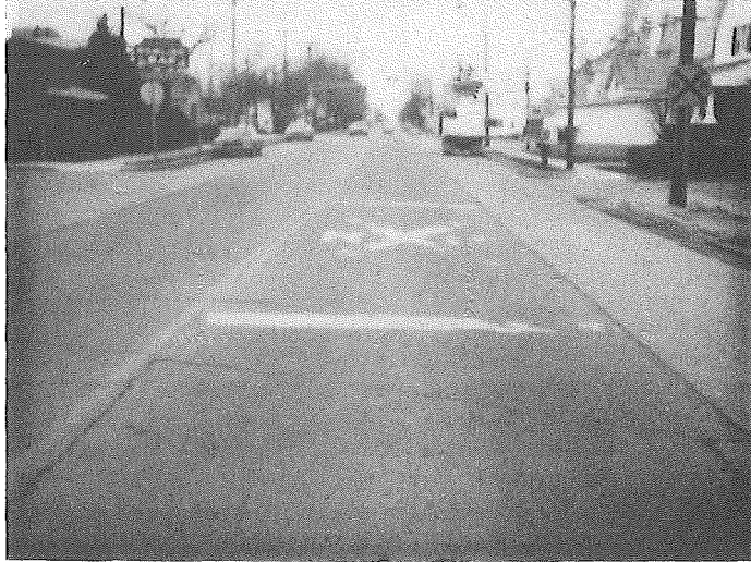
EB M-81 in Reese, Tuscola Co. Approximately 50% of the thermoplastic marking has disappeared. The pavement surface is good.
