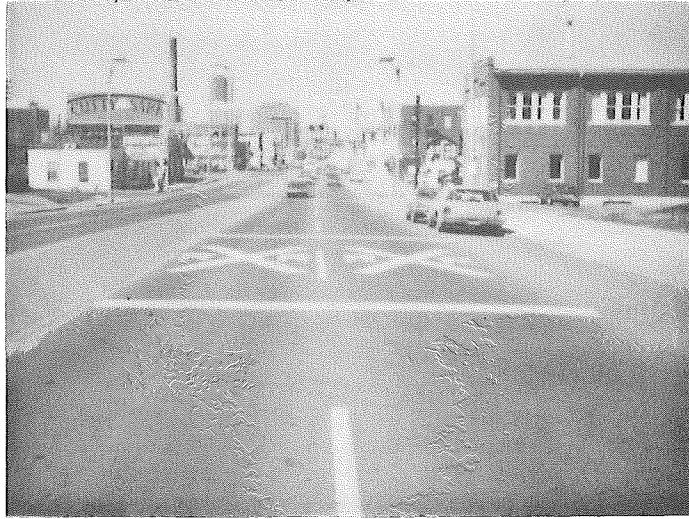
M-143 Michigan Ave. in Lansing The thermoplastic pavement marking is totally intact after one winter.
