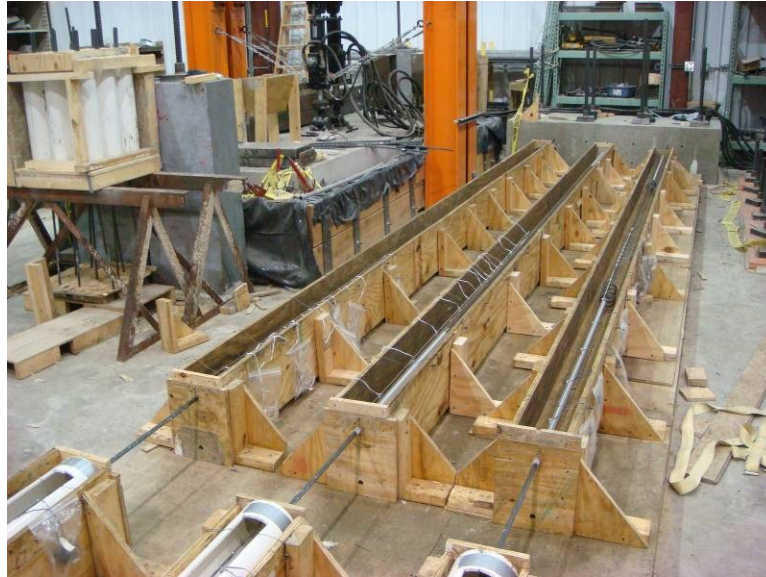
Figure 21 Form Work of Small Prestressing Concrete Beam Units
