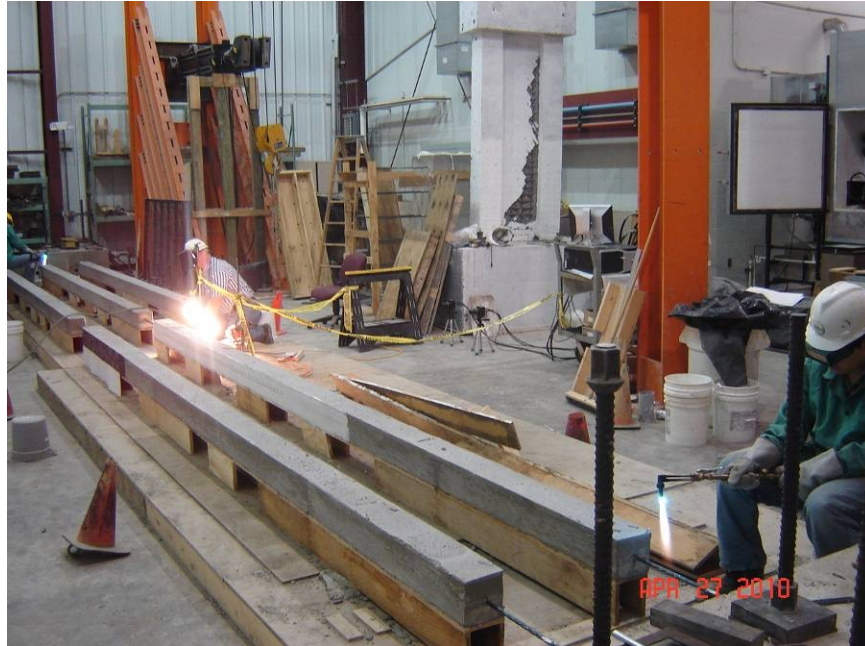
Figure 23 Releasing of Prestressing Strand
