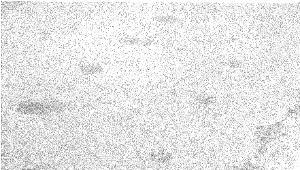
Figure 3. Typical core location.
