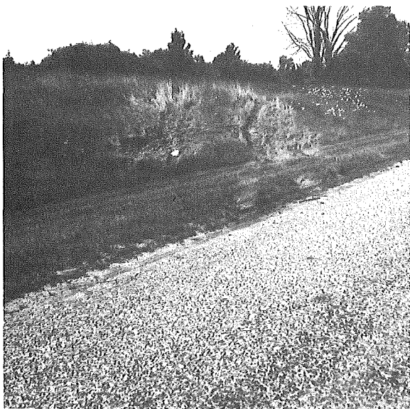
This photo shows a 1 on 4 back slope which an out-of-control vehicle struck while skidding sideways, causing the vehicle to overturn resulting in fatal injuries to the driver.
