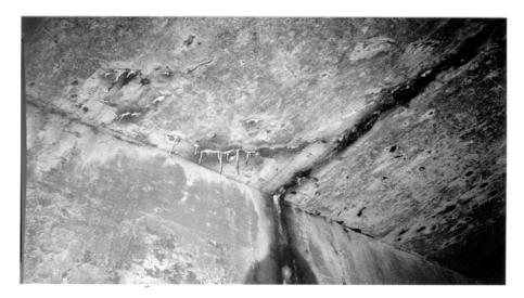
Figure 1 . Calcium carbonate deposits on underside of bridge deck.
