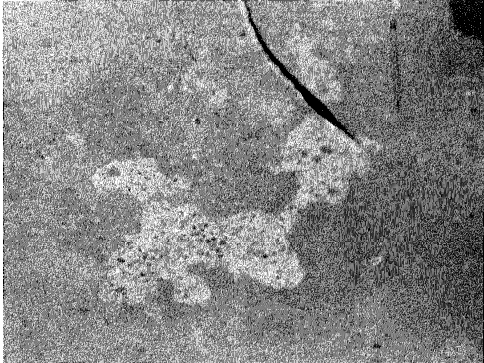
Figure 5. View of scaled area at Station 88+20.
