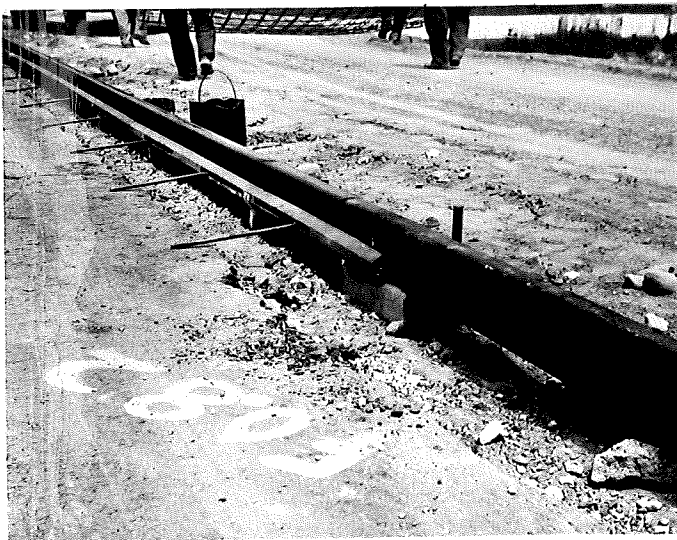
▲ FIGURE 12. VIEW SHOWING AN EXCEPTIONALLY GOOD METHOD OF INSTALLING TIE BARS.
