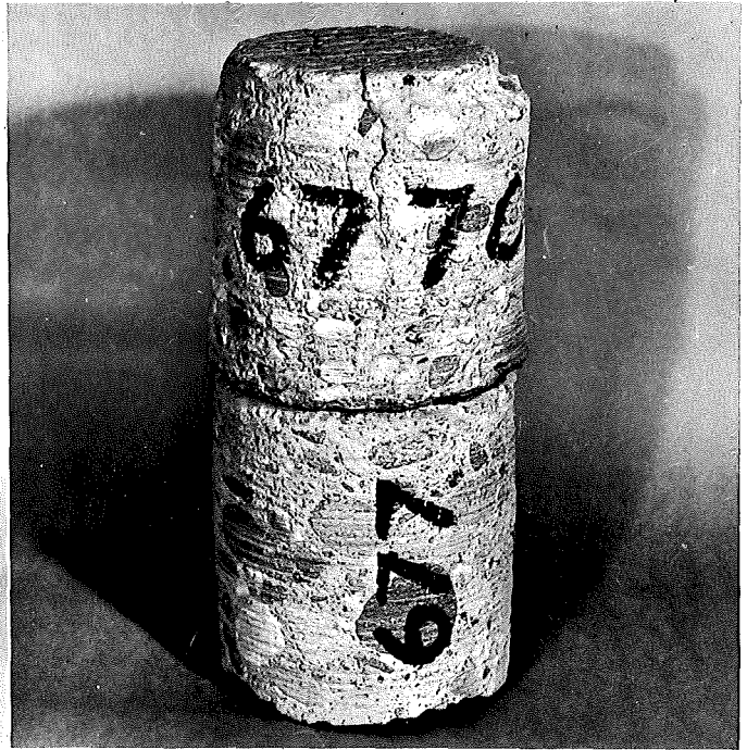
FIGURE 21. CORE TAKEN AT STATION 21 + 14 TO SHOW CRACK IN CAPPING BUT NO CRACK IN BASE COURSE UNDERNEATH THE CAPPING. DECEMBER 18, 1952.
