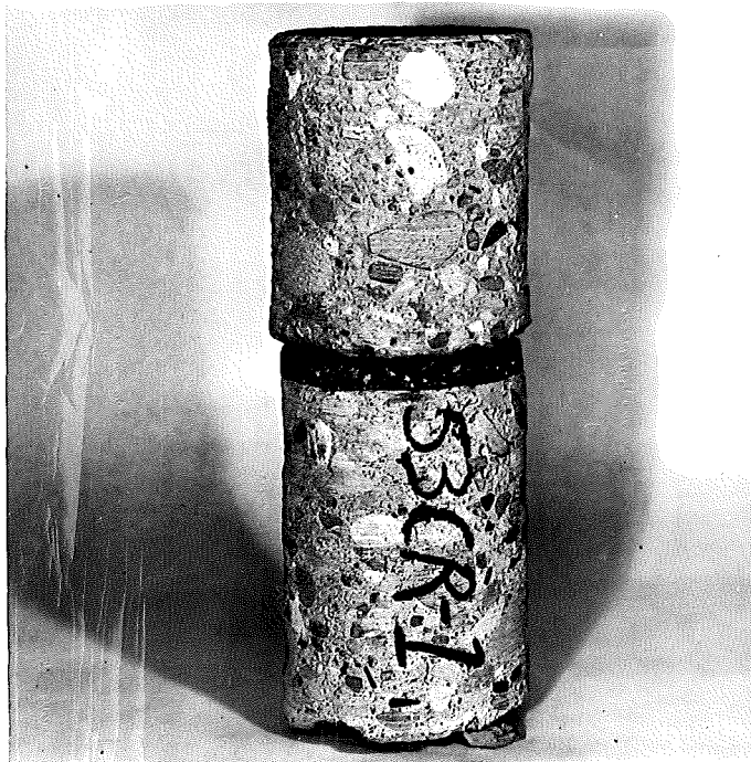
FIGURE 20. CORE SHOWING BITUMINOUS BREAKER STRIP BETWEEN OLD CONCRETE AND CAPPING CONCRETE. STATION 289 + 00. JANUARY 16, 1953.
