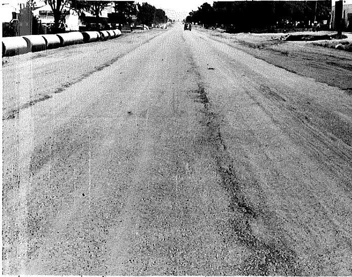
FIGURE 6. SURFACE OF EXISTING PAVEMENT IMMEDIATELY AFTER PLACING OF AE-3 AND SAND (STD. METHOD) NOTE THAT TRAFFIC IS BEING CARRIED. JUNE 27, 1952.
