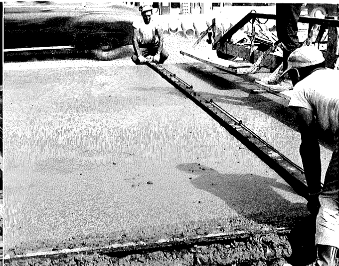
▲ FIGURE 15. PLACING TEMPLATES WITH GROOVING BAR IN FRESH CONCRETE.
