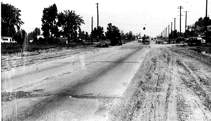
▲ FIGURE 3. VIEW OF ORIGINAL SURFACE BEFORE CAPPING. STATION 119 IN SECTION WHERE 7" CAPPING WAS PLACED USING REGULAR METHOD OF A E - 3 AND SAND. JUNE 13, 1952.
