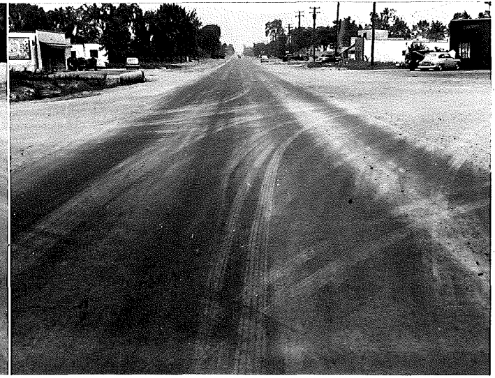
FIGURE 9. LOOKING NORTH FROM STATION 250 SHOWING 3/4" BITUMINOUS CONCRETE BREAKER STRIP IN PLACE. JUNE 13, 1952.
