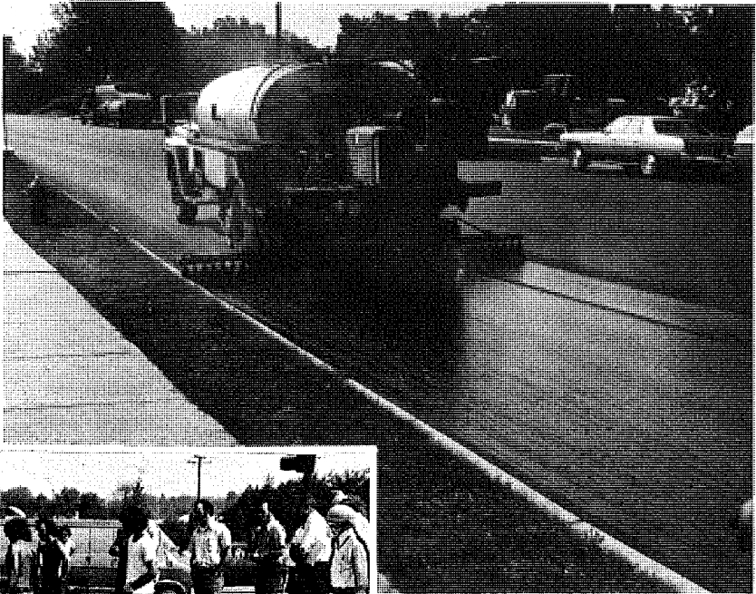
Figure 4. Placing Petro-mat fabric with roller mounted on the front of an Allis-Chalmers tractor and stiff bristle attempting to smooth it behind roller. Unrolling each 300-ft roll, 12-ft wide, took 15 to 25 minutes.
