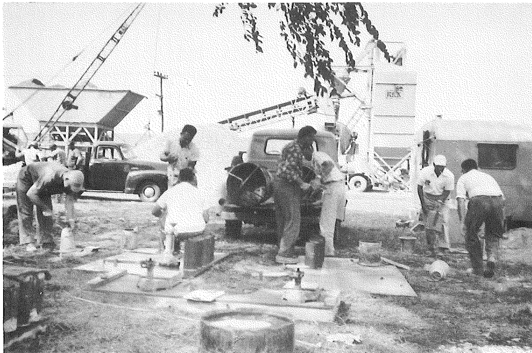
Figure 4. Testing site with batch plant in background.
