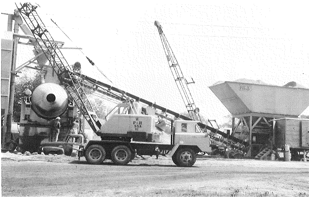
Figure 2. Mixer, traveling crane, belt conveyor, aggregate bin, and control house.
