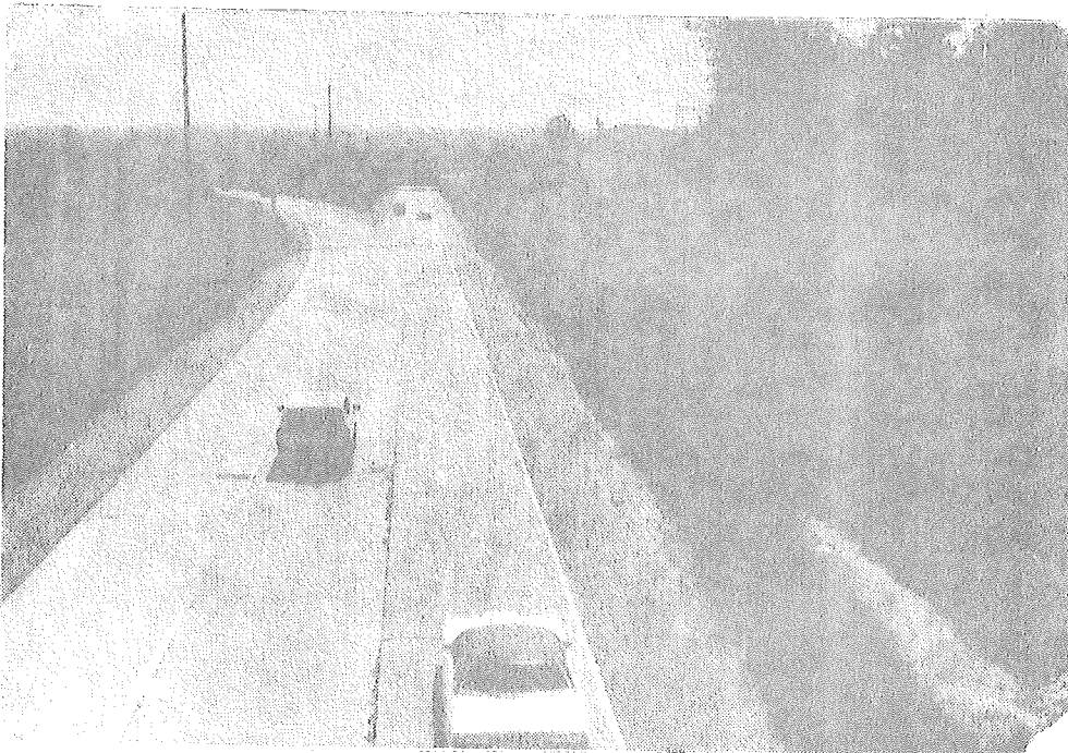
Figure 6. Looking easterly (from the M-37 overpass) at downstream location.
