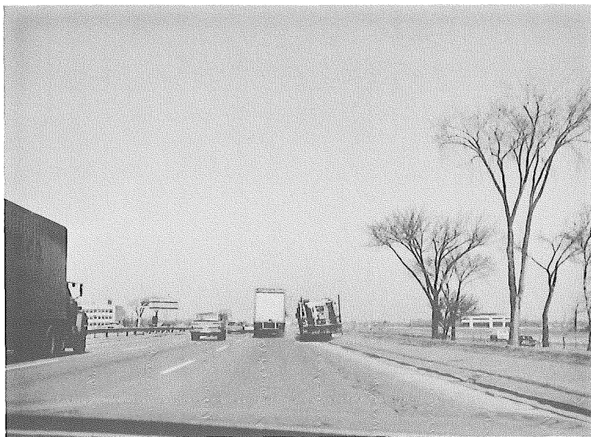
Photo 5 - An example of the merging conflict on the northbound Southfield Freeway. The auto hauler attempting to merge onto the freeway from the entrance ramp is forced onto the shoulder by 100-foot truck.
