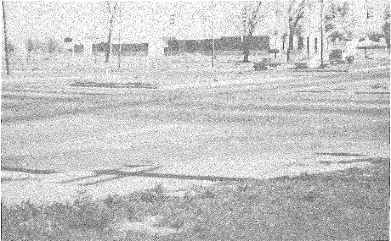
Figure 20. Sand-asbestos surface, 4 years after construction showing raveled fillets.
