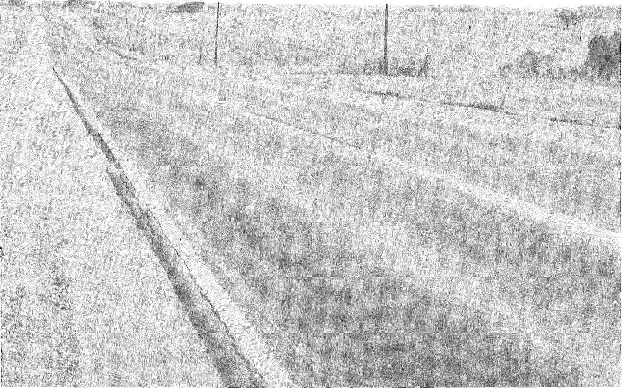
Figure 13. Sand-emulsion surface, 4 years after construction.
