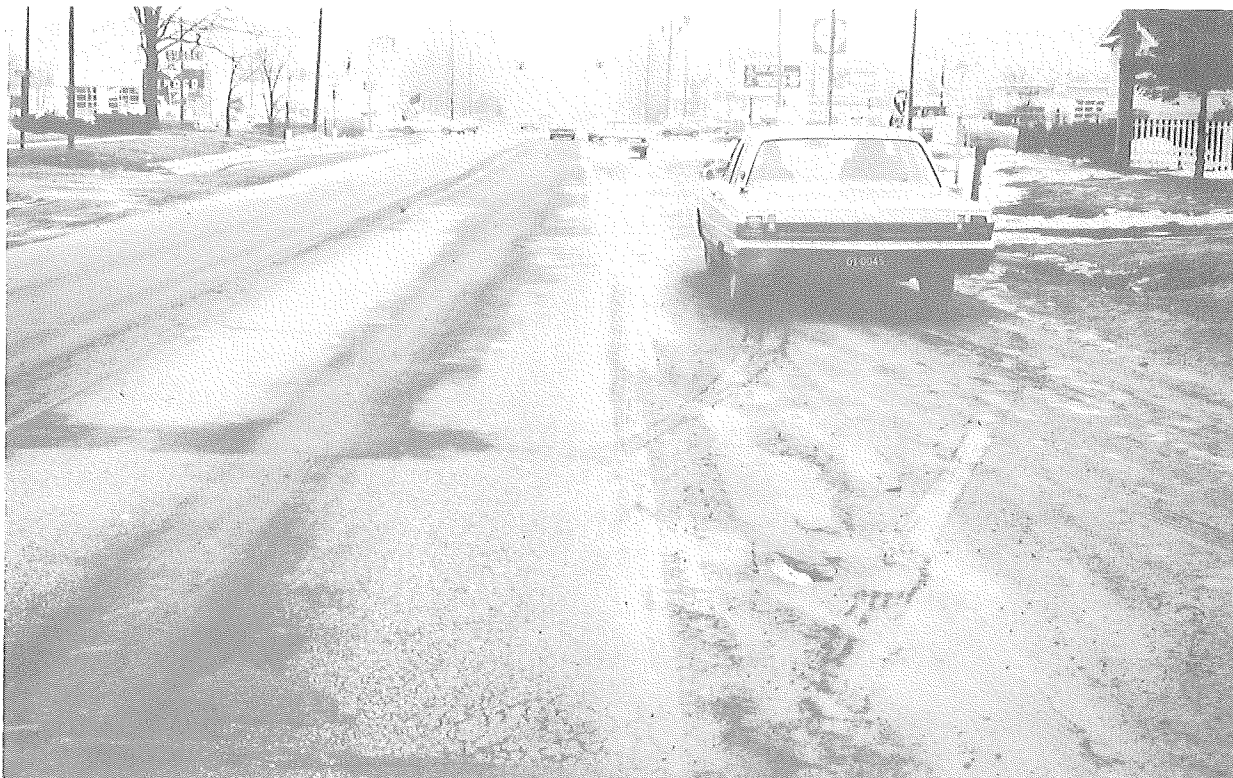
Figure 11. Crushed trap rock, 3 years after construction.
