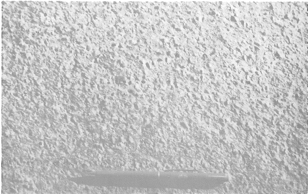
Figure 10. Close-up of beach pebble surface, 4 years after construction.
