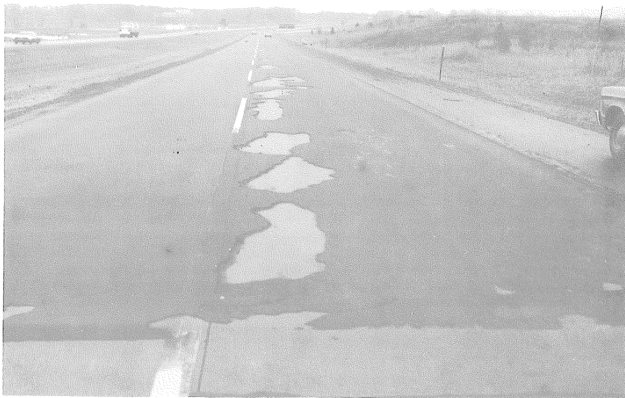
Figure 12. Synthetic bitumen and sand, 1 year after construction.
