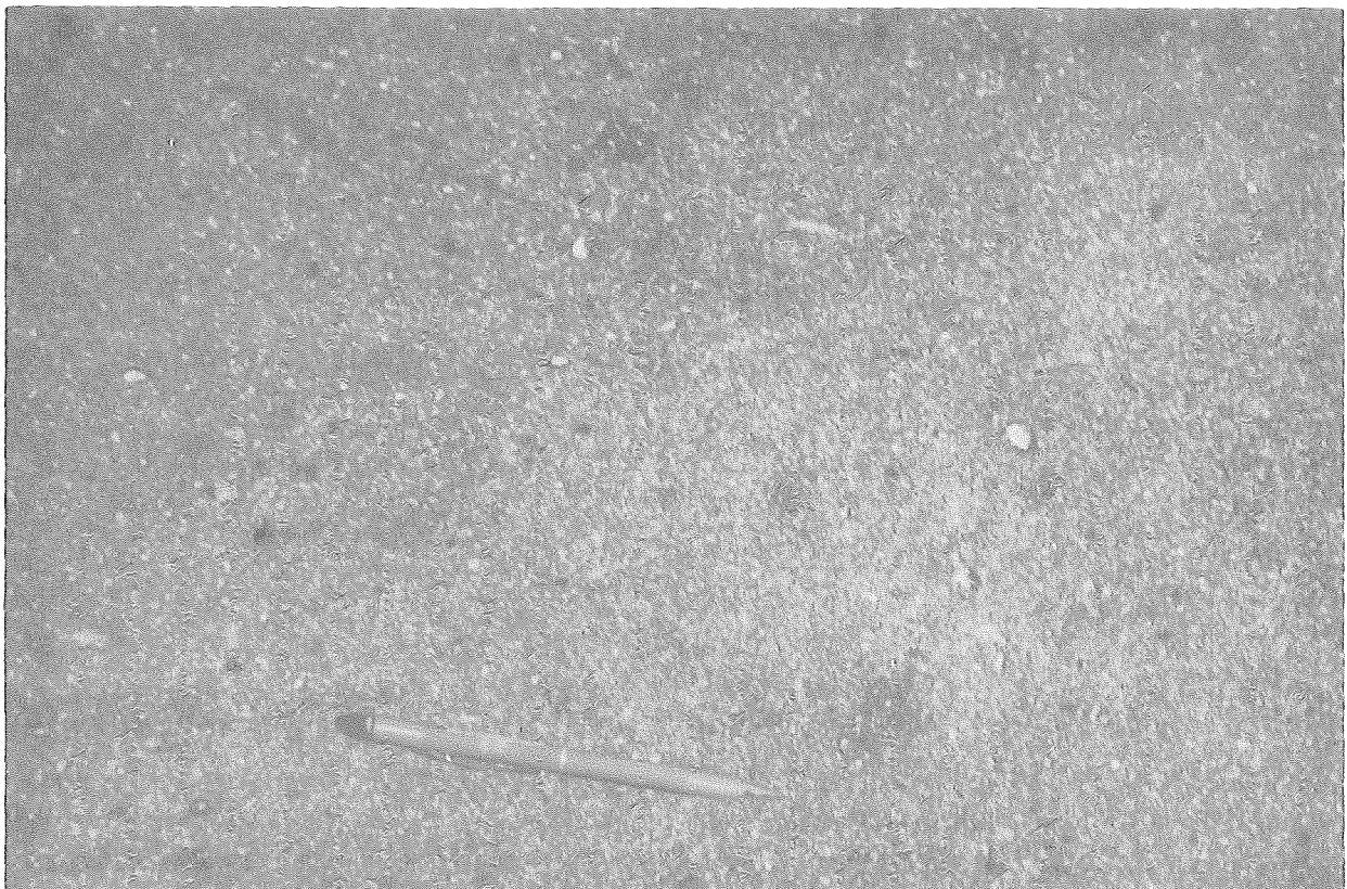
Figure 21. Close-up of sand-asbestos surface, 4 years after construction.
