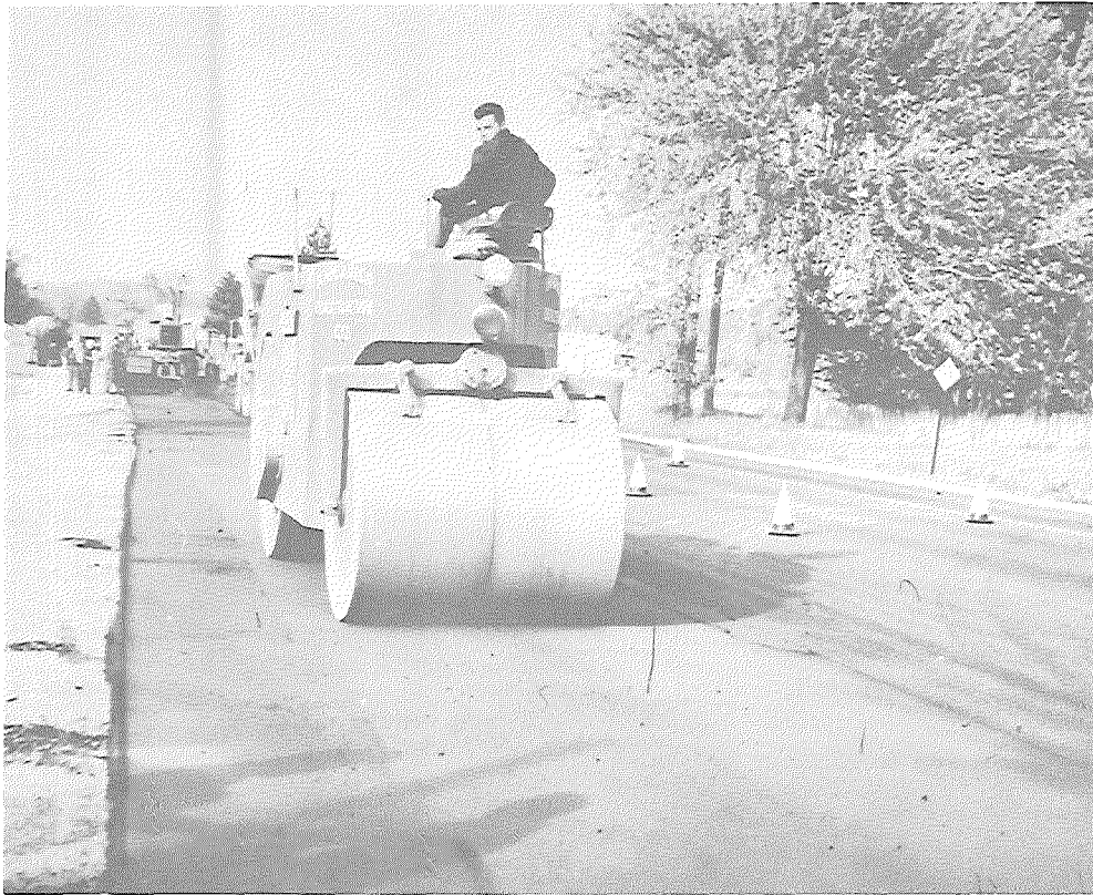
▲ Figure 29. Rolling pavement after sand application.
