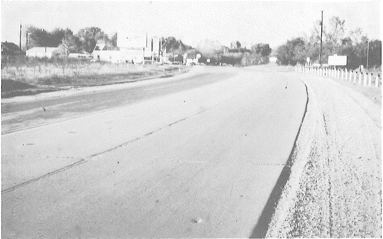
Figure 22. Synopal-sand surface, 4 years after construction.
