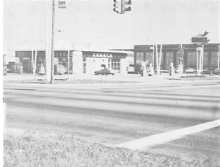
Figure 18. Stone-filled sand-asphalt surface, 4 years after construction.
