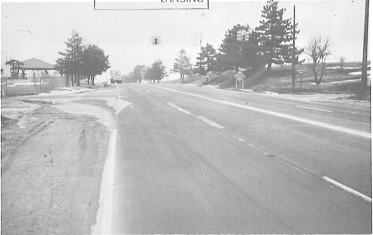
Figure 7. Crushed quartzite surface, 3 years after construction.
