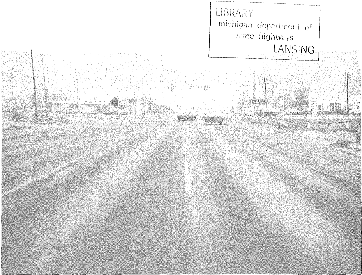
Figure 9. Crushed beach pebbles, 3 years after construction.
