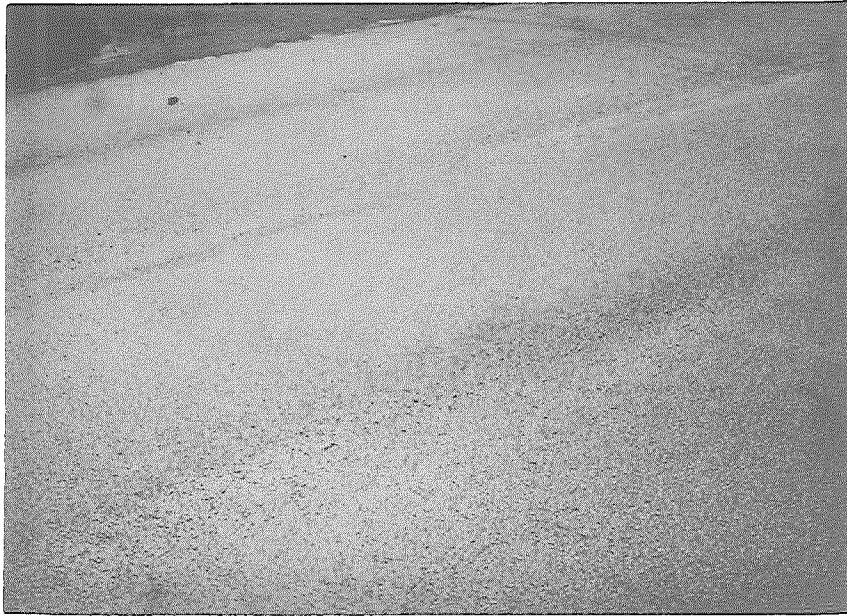
Figure 1. Polished limestone-slippy pavement surface.
