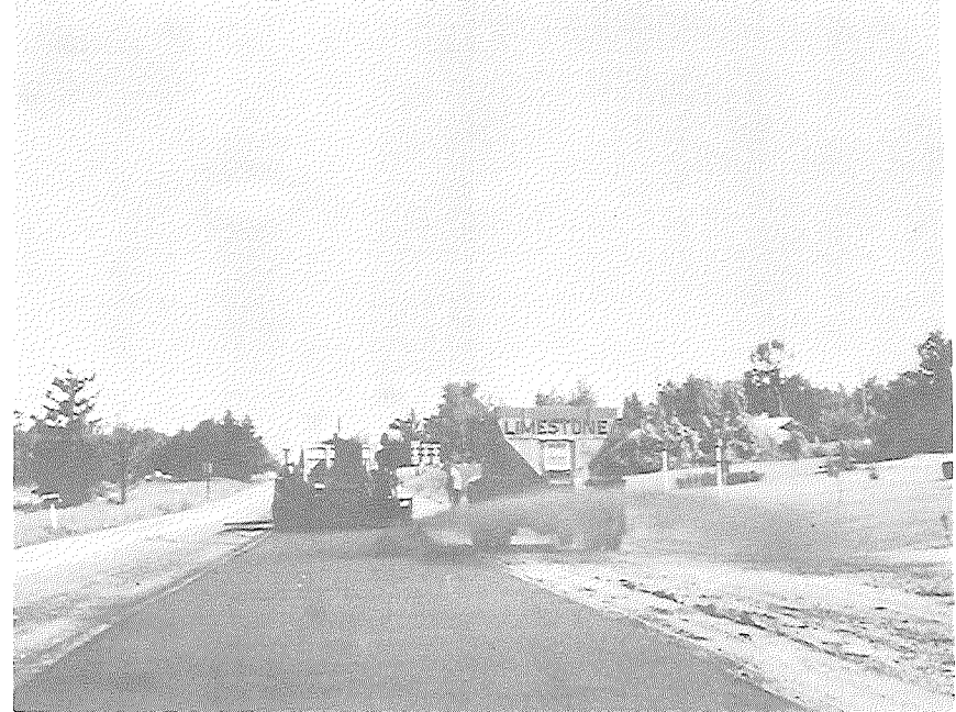
Figure 27. Spreading precoated sand - showing sand being wasted on shoulder.
