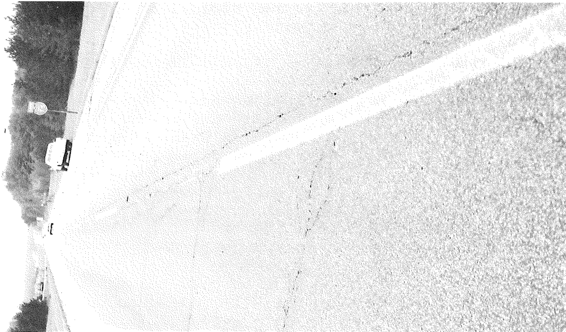
Figure 2. Typical distress conditions of the original 15-year old flexible pavement, construction Project I 69014-09240A on southbound I 75 about 10 miles north of Gaylord in Otsego County.
