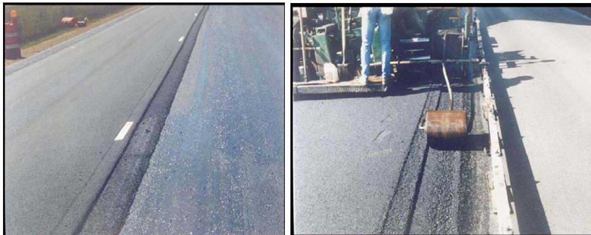
Figure 8. Notched Wedge Joint (a small steel drum is attached to paver to roll the wedge behind the paver)
