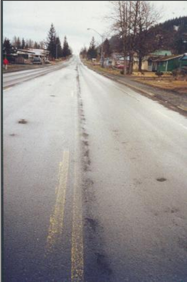
Figure 1. Photograph Showing an Example of Accelerated Deterioration Along a Longitudinal Centerline Joint that was Inadequately Constructed
