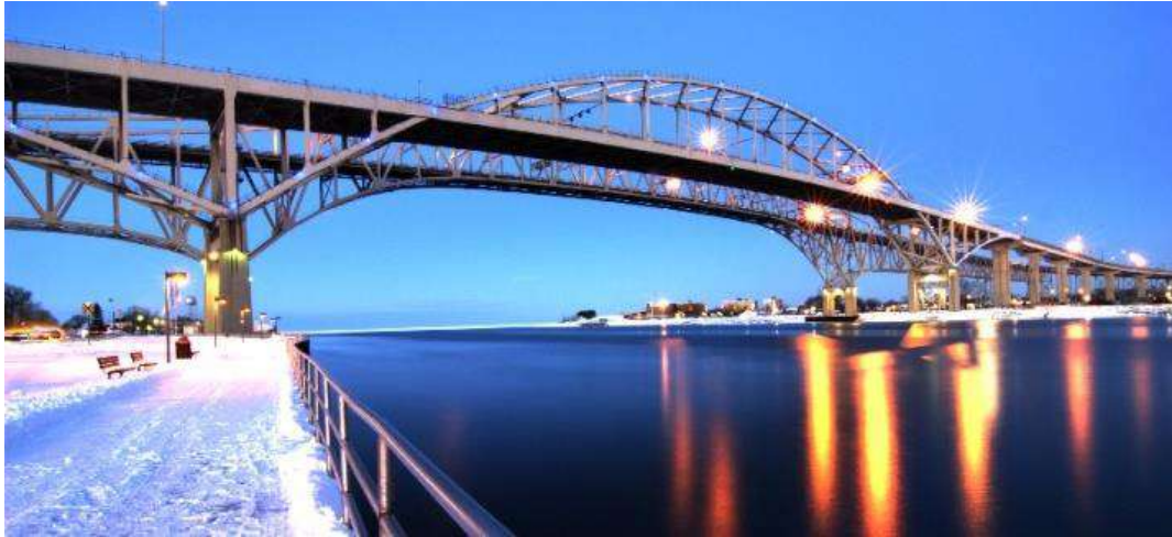
Figure 4.16 - Blue Water Bridges between the USA (Port Huron, MI) and Canada (Sarnia, ON).
