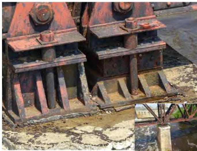
Figure 1.14 - Example of high resolution photography in difficult to access locations obtained with UAV. From Zink and Lovelace (2015).
