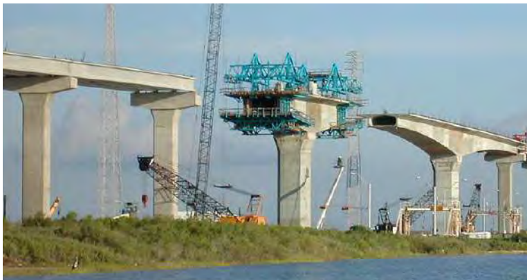
Figure 2.6 - View of Quintana Beach Bridge under construction in Texas.
