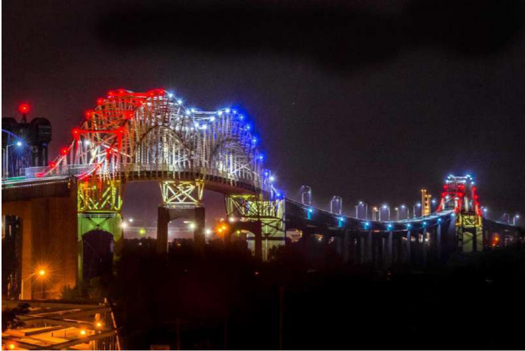
Figure 4.40 - Sault Ste. Marie International Bridge.
