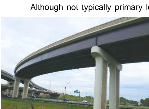
Figure 4.7 - Curved girder bridge
