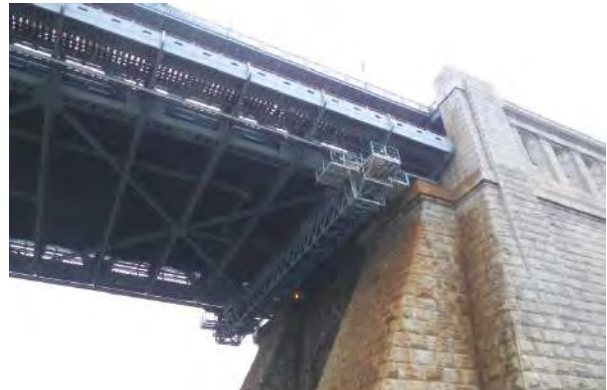
Figure 2.2 - View of motorized traveler system used on the Benjamin Franklin Bridge.
