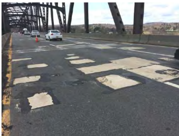
Figure 2.10 - Repair patches in the deck of the North Newburgh-Beacon Bridge.
