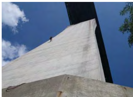
Figure 4.1 - Inspector rappelling a reinforced concrete pier tower.
