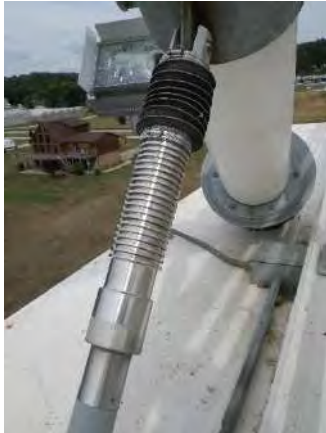
Figure 4.9 - Stay Cable Vibration Dampener
