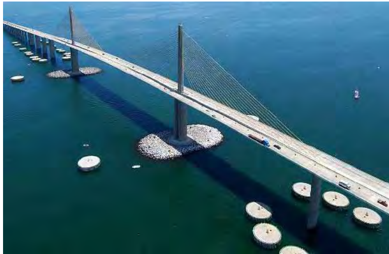
Figure 4.10 - Numerous dolphins and placed riprap protecting the Sunshine Skyway Bridge.
