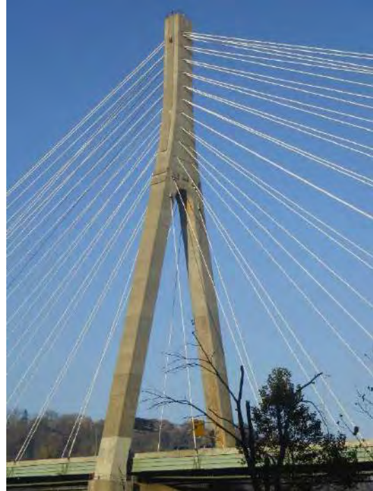
Figure 4.11 - Veterans Memorial Bridge, West Virginia.
