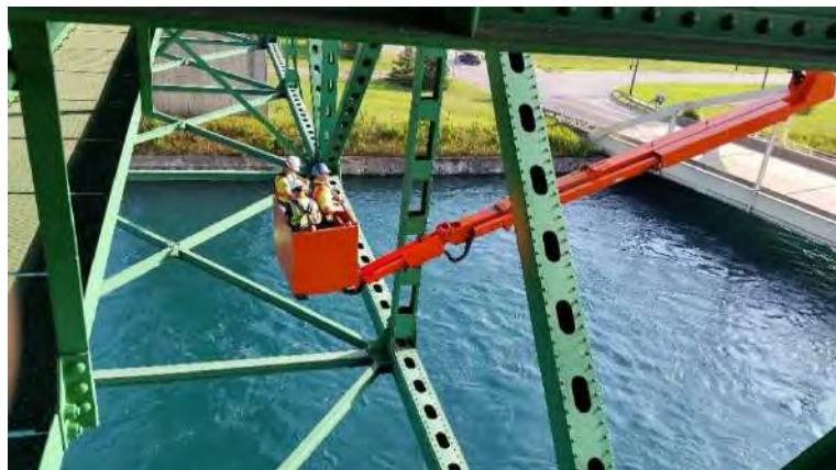
Figure 4.17 - Inspectors in an underbridge inspection unit (UBIU) inspecting a deck truss.
