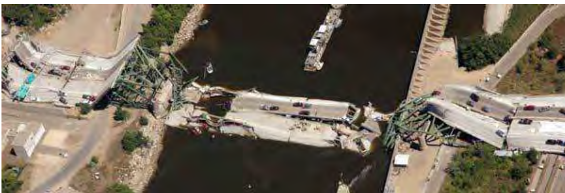
Figure 1.4 - Aerial photograph of the collapsed bridge deck truss sections of the I-35 W bridge after the collapse. (MnDOT 2008).
