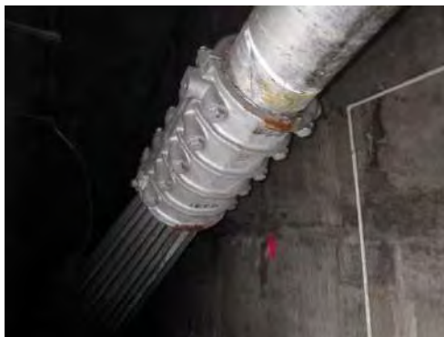
Figure 4.3 - Steel main cable splay casting.
