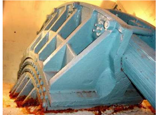
Figure 4.4 - Steel main cable tower saddle.
