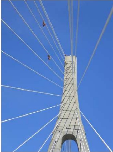
Figure 2.3 - Inspectors using technical rope access techniques.
