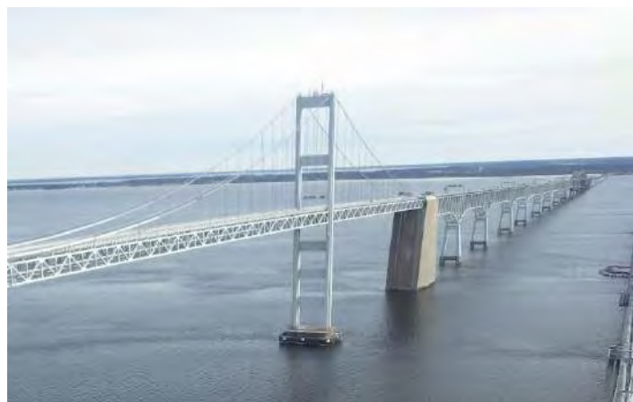
Figure 4.14 - Suspension and cantilever truss sub-units of Westbound Chesapeake Bay Bridge.
