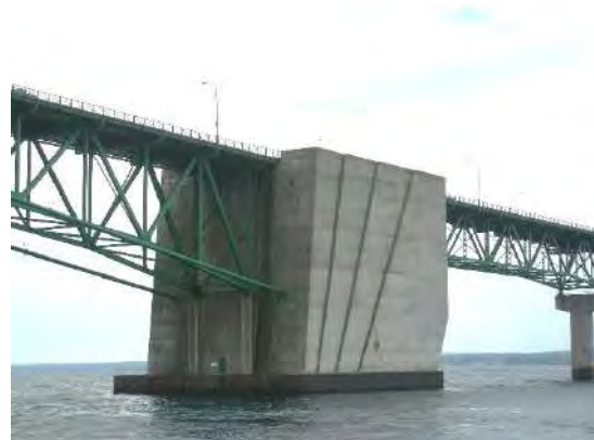
Figure 4.2 - Reinforced concrete anchorage chamber on the Mackinac Bridge.
