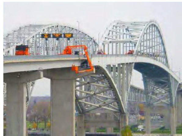
Figure 2.5 - Second Blue Water Bridge being inspected with a UBIU.
